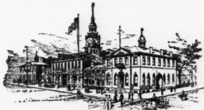
Old Independence Hall, covered with Taylor's "OLD STYLE" Brand Tin.
