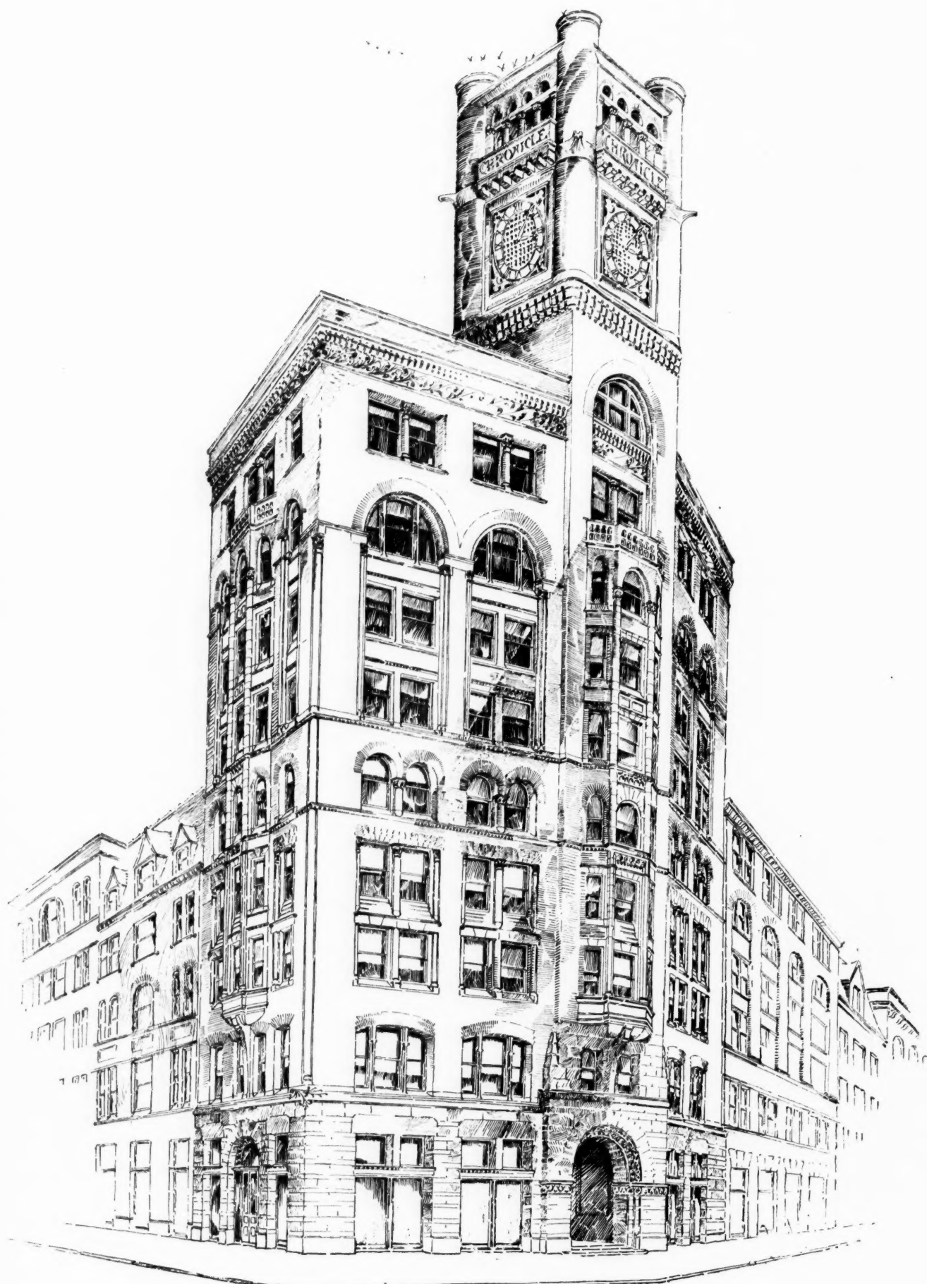
THE CHRONICLE BUILDING, SAN FRANCISCO, CAL.
