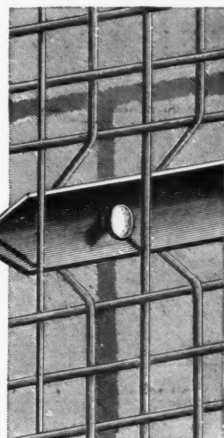
Full size of Lathing secured to brick wall.
