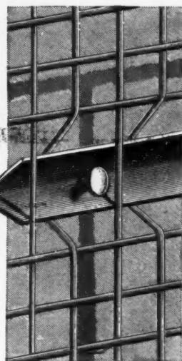
Full size of Lathing secured to brick wall.
