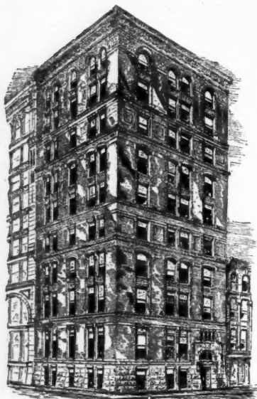
COUNSELMAN OFFICE BUILDING, CHICAGO. Burnham & Root, Arch'ts.
