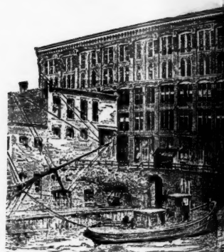
HIRAM SIBLEY WAREHOUSE
