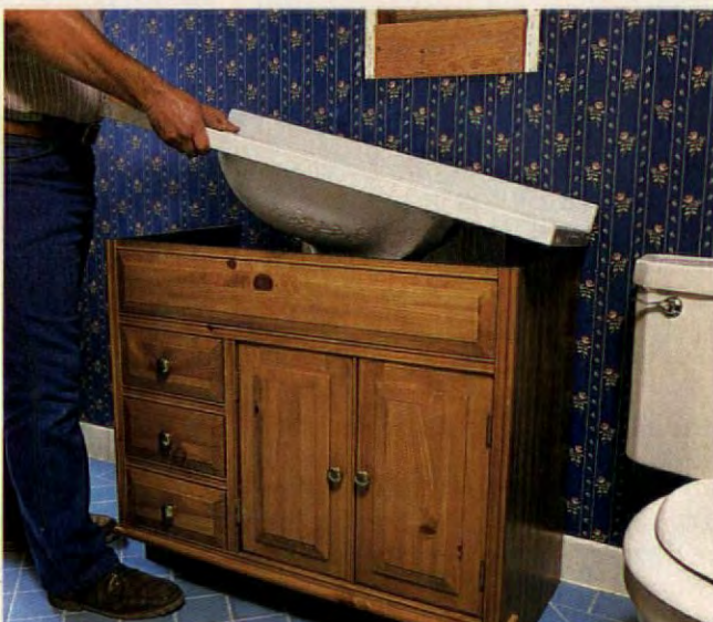
Place new sink top and vanity in position. Make sure top is centered and overhangs sides and front of vanity equally.
