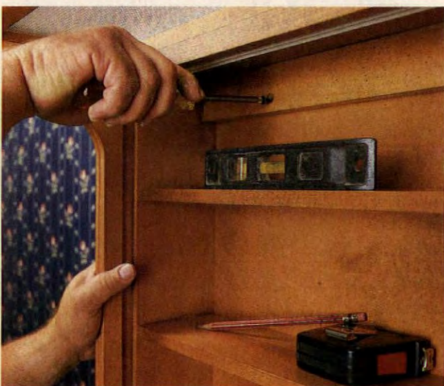
Screw the leveled medicine cabinet into a wall stud; you'll need a helper. Switch off electricity before connecting any lights.
