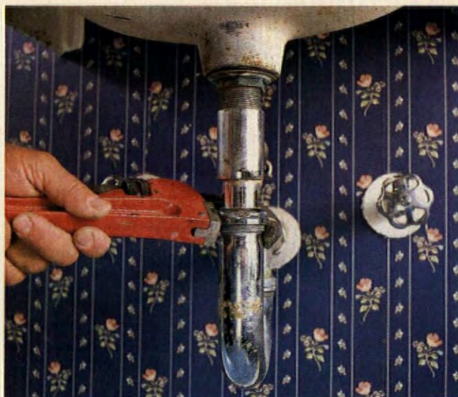
Loosen coupling nuts on J-trap with pipe wrench or locking pliers. Trap will have water in it, so have a bucket handy.
