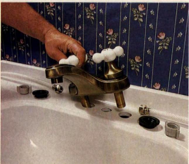
Slide faucet shanks into sink top, tighten with flanges from below and connect to shut-off valves with new supply lines.
