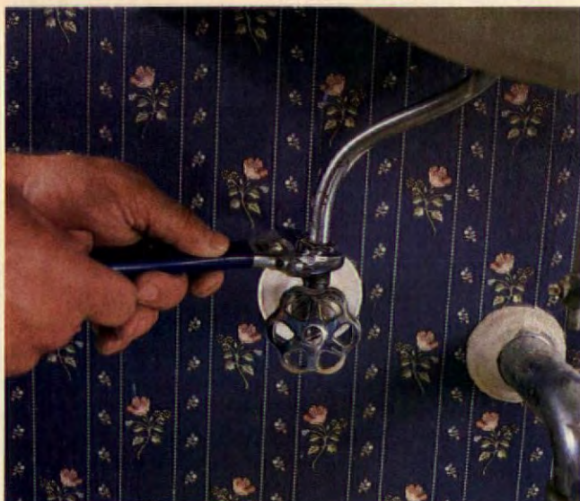
Disconnect water supply lines after closing shut-off valves or main water line to house. If valves are old, replace them.
