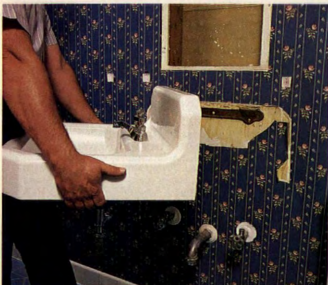
Lift sink up off its bracket with care; it will be heavy. Unscrew bracket. Note cavity of old cabinet; new one will cover it.
