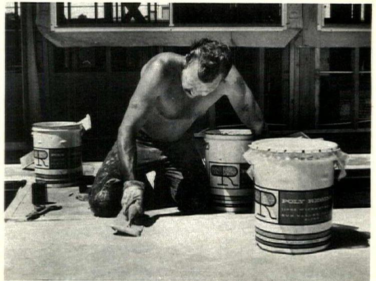
**Polyurethane skin** is both a seamless waterproof roof coating and a durable deck. It covers concrete (foreground) or plywood (background). Consistency for spraying,
