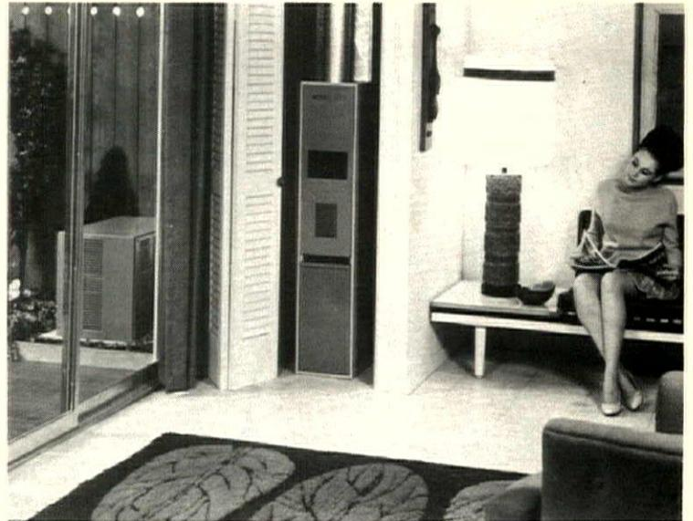
**Compact furnace** for apartments or smaller homes is only 11" wide, 52" high, and 28" deep and will fit into a closet. The gas-fired furnace, teamed with a cooling coil,
