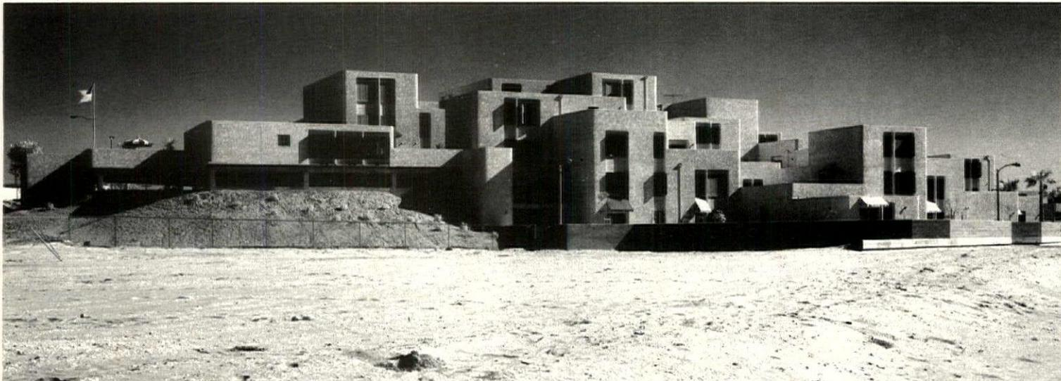
Beachfront apartment is planned on 22-ft. modular grid. The result is planned irregularity in the five-level facade. Sea wall protects front.
