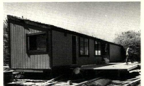
**Construction photos** show box sitting on temporary foundations of screw jacks (*above*). Running gear is permanent on these models, but on most houses it is removable. Unfinished interior (*below*) shows abutting ridges and posts ready to be bolted together and cased.
