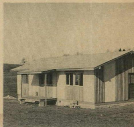
**EXPERIMENTAL HOUSE** in Kentucky was built by four unskilled workmen with color coded jigs.
