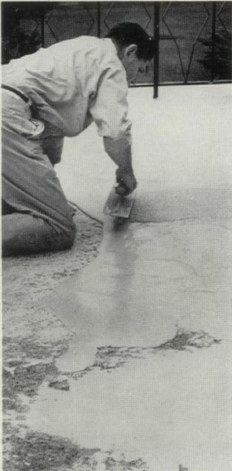
**THIN COAT** of silicone topping—usually  $\frac{1}{8}$ " thick—is troweled on for \$1.00-\$1.75 per sq. ft.
