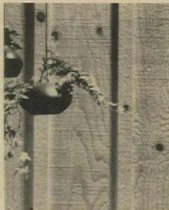
**Plywood siding** of white pine has a rough-sawn surface. Trend-Tex siding is available in six factory applied stain finishes with battens or decorative grooves. The surface is treated with a water repellent preservative. Potlatch, San Francisco.
