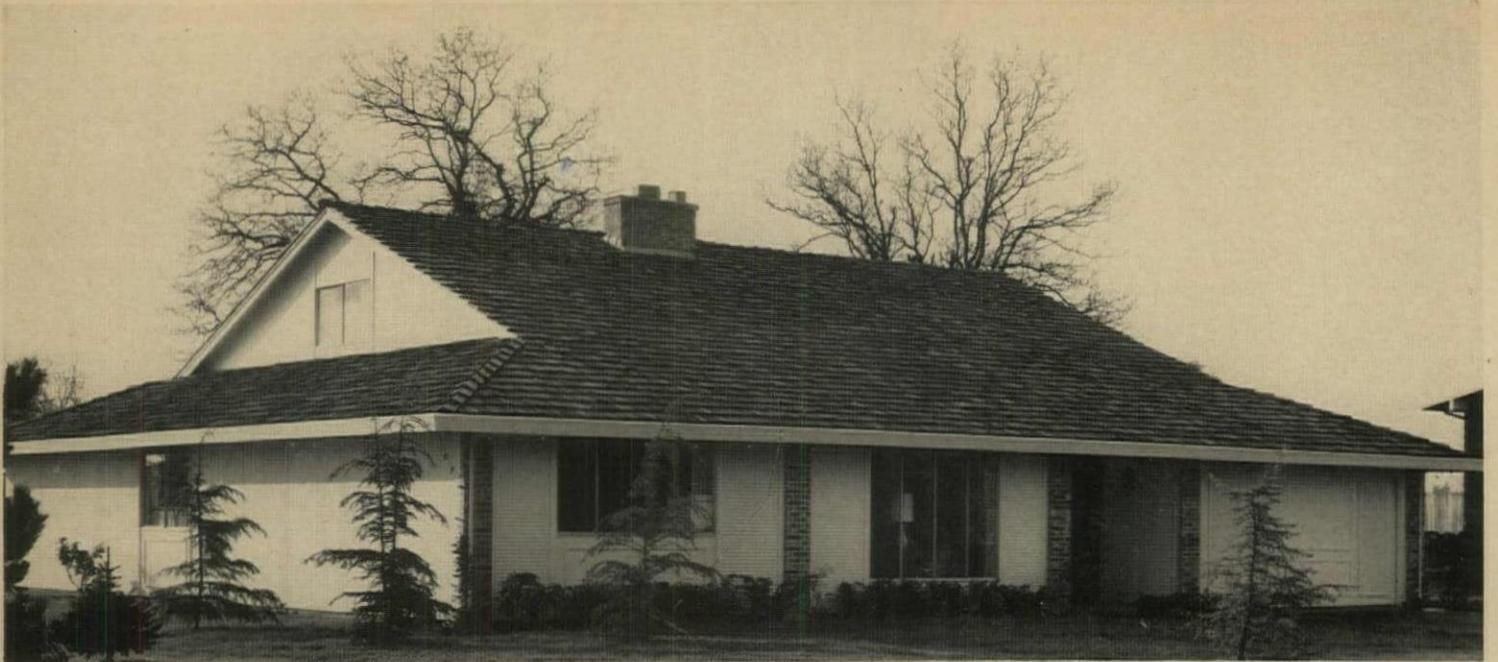
**SIMPLE RECTANGULAR SHAPE** of 2,500-sq.-ft. house is key to its low cost. Wall area is the same as on an L-shaped ranch of about 1,800 sq. ft.
