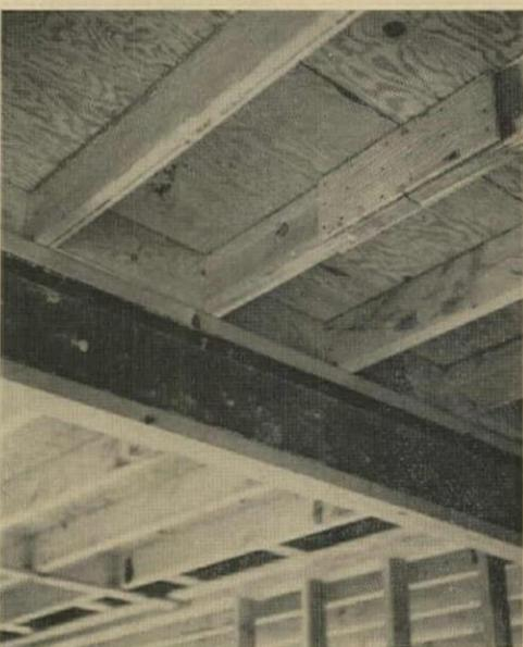
**FLOOR SYSTEM** of in-line joists demonstrates strength of glue-nailed splice joints and ability of 2x6 members to perform as well as 2x8s when
