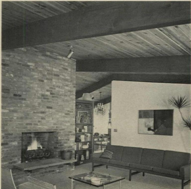
**PLANK-AND-BEAM CEILING**, shown here in the living room, is uncluttered because wiring for overhead fixtures runs through chases routed in the roof.
