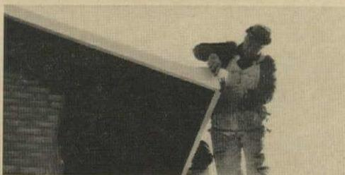
**BUILT-IN GUTTERS** are constructed around continuous 2x8 nailed to rafter ends and interlocked with roof sheathing. This serves as rain stop and
