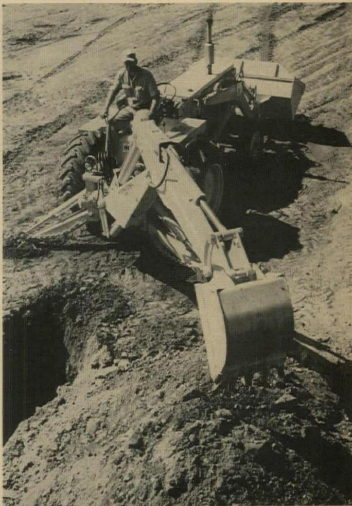
**Hydraulic-cushioned backhoe** digs to 12½', operating at 2,100 psi. It has full feathering control and simultaneous crowd, lift and curl action. Two other models dig to 14' and 15'. Bucket widths: 12" to 36". Int'l Harvester, Chicago. (Circle 218 on Reader Service card)
