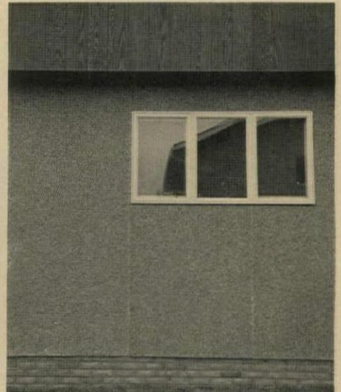
an exposed seam (above) between 4"-wide panels, but manufacturer supplies a touch-up kit of matching aggregate to avoid use of batten strips.
