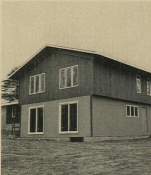
**PLASTIC-CLAD WALLS** and windows practically eliminate outside maintenance. Factory-applied aggregate-on-epoxy finish on lower walls leaves
