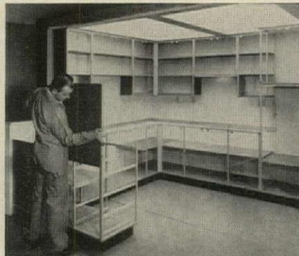
**PANELS** slip into grooves formed in frames.
