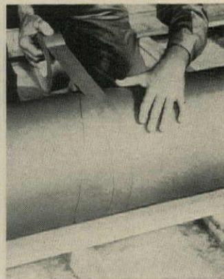
SECTIONS ARE JOINED with a metal sleeve, then sealed with tape.
