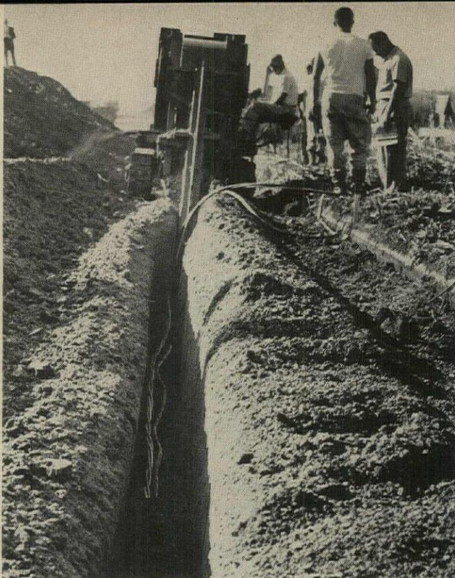
**TRENCHING** can usually be done cheaper by builder than utility—builders' costs run as low as 10¢ a foot if job is lumped in with other earthmoving work. Job shown is Centex Construction at Elk Grove, Ill.
