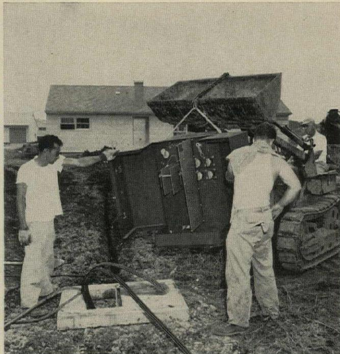
**PLACING TRANSFORMERS** is a job easily handled by builders' crews using standard equipment, so there need be no special installation cost. Hook-up is made by utility. Note trench for secondary line to house.
