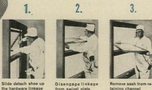
1. Slide detach shoe up the hardware linkage
