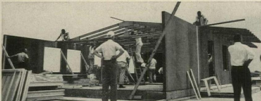
**ROOF TRUSSES** are put up on panel walls. End panels were left out until all trusses were up. Despite newness of the system, building crew closed in the house in one day.
