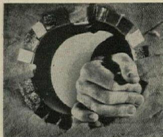
LATERAL JOINT is made over a sheet metal union.
