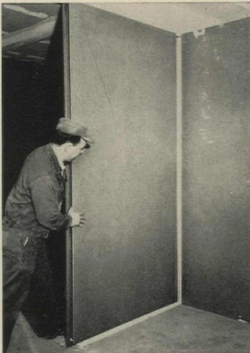
**UNFINISHED PANEL** is set against exterior wall. Skin has no nail dimples, so only joints need finishing.
