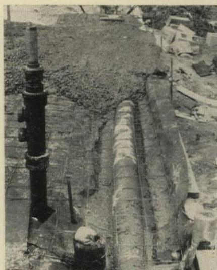
**7.** Monolithic pour forms slab and ducts at same time. Resulting jointless duct cannot be blocked with concrete or rubble.
