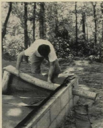
**2.** Forms are laid on vapor barrier, inflated to 14 psi. To turn corners, forms can be bent to a radius five times their diameter.
