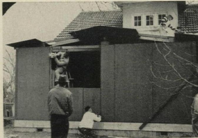
**ROOF IS SHEATHED** and picture-window frames set in place. Total time for the whole job, including trim and roofing: 7½ hours. /END
