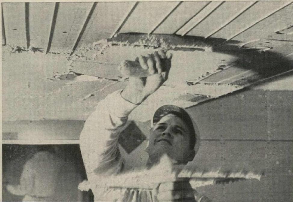
**SIMPLE TO INSTALL**, heating cable is completely covered by ceiling plaster. No time is lost, because the electrical subcontractor handles electric heating along with the rest of his wiring job. And the Valentines like the fact there are no vents to cut.
