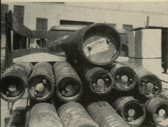
**ALUMINUM ENDS** of inflatable forms have tire-type valves. Forms can be used in any weather and stored in the open.
