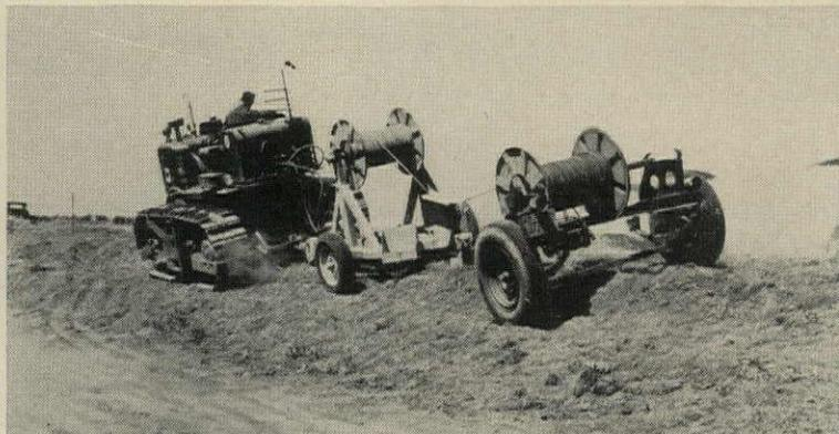
**CABLE-LAYING TRAILERS** are towed behind plow (left) which is pulled through earth by tractor. Cable is fed through the shoe of the plow to the correct depth, which is established by plow adjustments.
