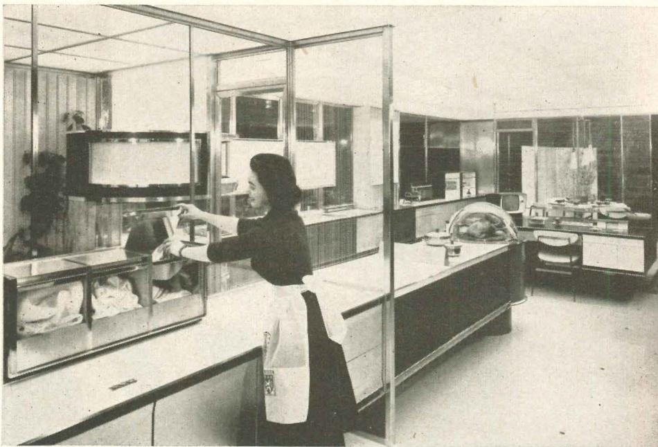
**Laundry** consists of three automatic compartments to sort fabrics by types. When any load reaches 8½ lbs., it slides over to washer. Washing time, temperature are selected automatically.
