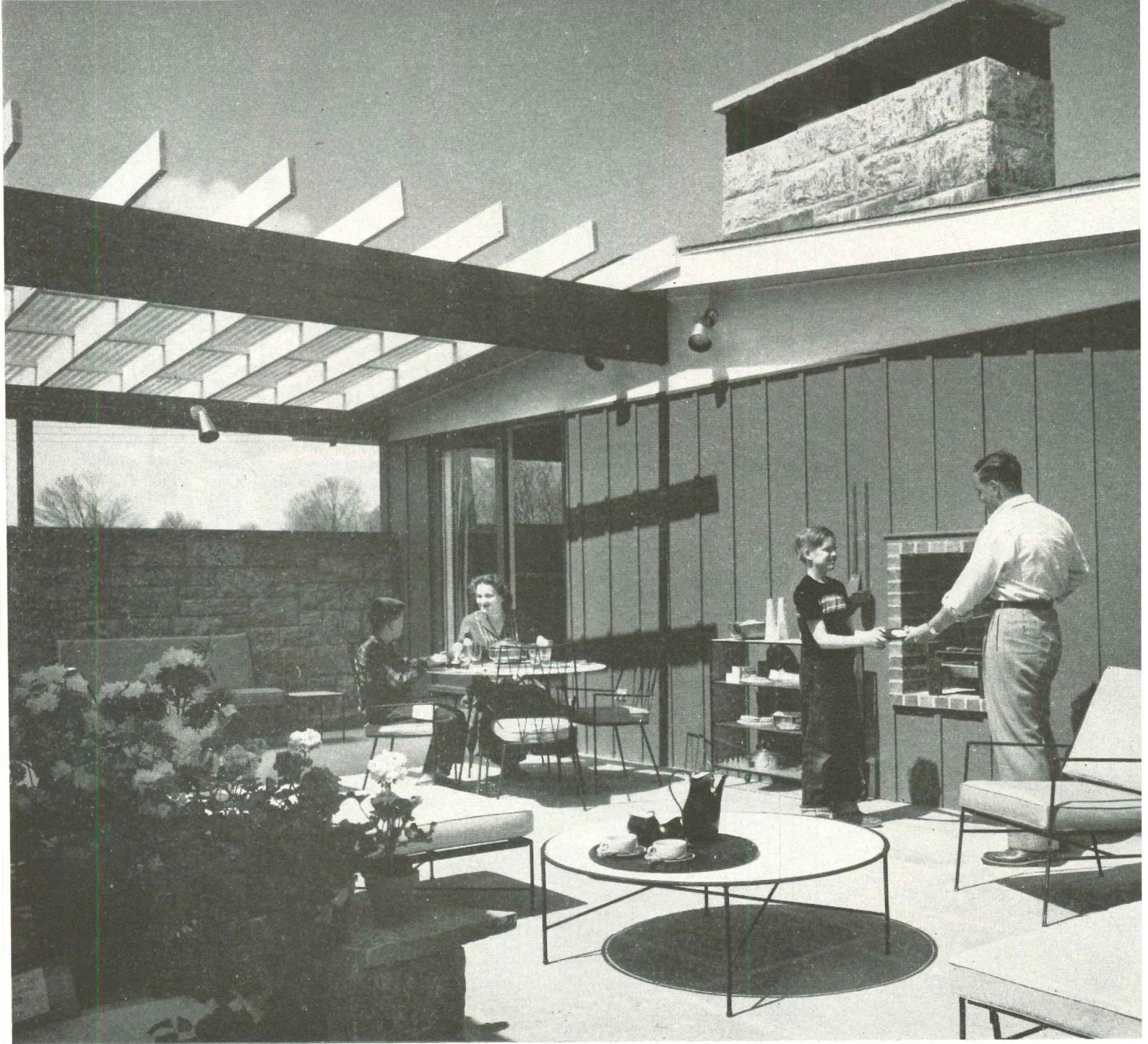
Colored plastic sheets cover the half of the terrace which leads carport and tool house to double glass doors of dining and kitchen. Rafters and plastic in pilot model cost \$450. Builders were unanimous in approving this terrace and its placement. Elaborate view above gives three way use for living, eating and cooking.
