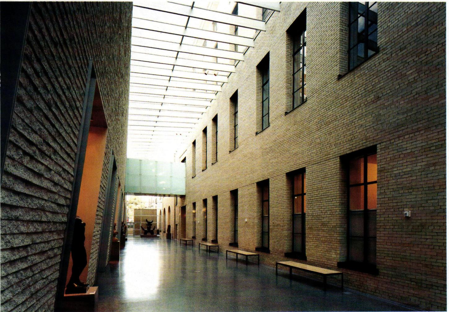
The brick rear wall of the landmark 1927 structure forms one flank of the new spine around which the Perelman Building is arranged. Split concrete blocks front new galleries for photography, costume, and modern design.
