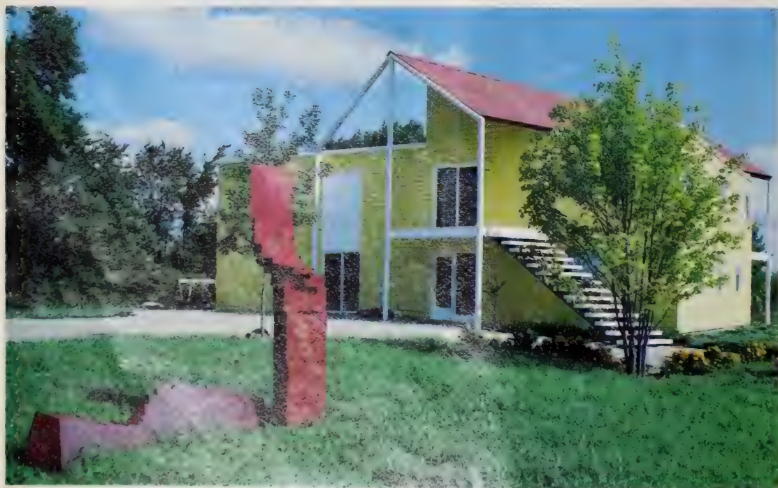
Looking like a Midwestern farmhouse lifted by a cyclone and then set back down a bit askew, the Barr house contrasts familiar architectural forms—pitched roof, front and back porches—and modest building materials—buttercup-yellow wood siding, red-painted corrugated-metal roofing—with a startling configuration that serves as a double entendre for the sculptures on the lawn are by the owner.
