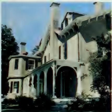
Front of house, top, was remodeled in neo-Georgian style in 1916 by the fashionable New York firm of Delano and Aldrich (architect William Adams Delano was a cousin), while rear, above, was frugally left in original Victorian style. Core of the house dates to the early 1800s.
