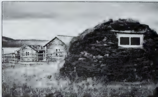
Adaptation to extreme winters: a cottage in northern Lapland covered with thermal layers of soil.
