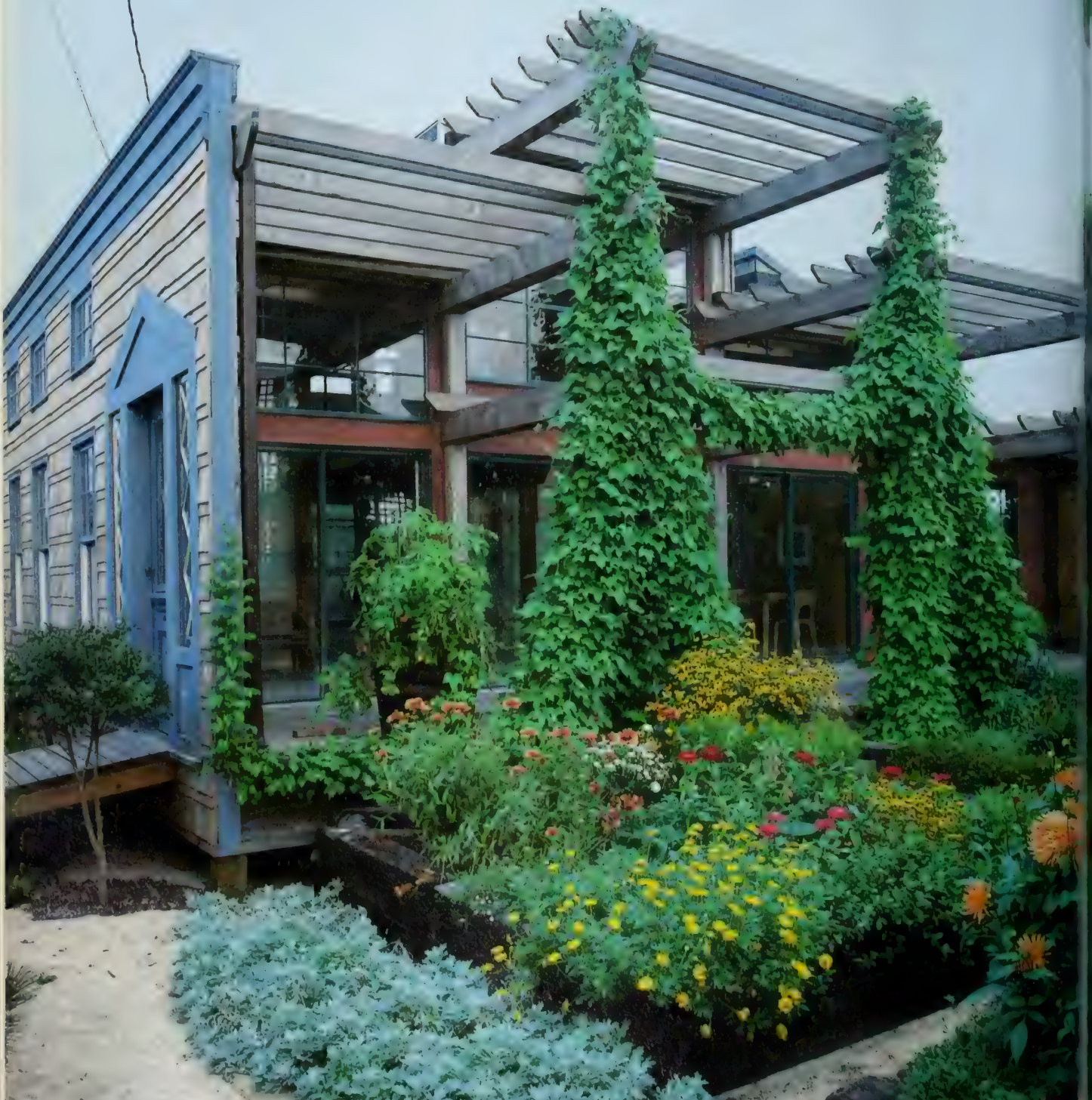
T he Fire Island, New York, house, above, designed by architect Peter Wilson, is a playful exercise in spatial illusion. The garden pavilion, opposite page, mimics the house: Its "windows," spiral staircase, and projecting bay echo identical elements on the far side of the main structure, making the pergola appear as though it were pulled away from the house.
