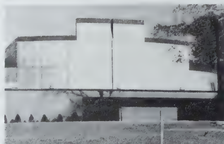
□ Exterior of the C.W. Post hall is clad in pewter-colored aluminum paneling.
