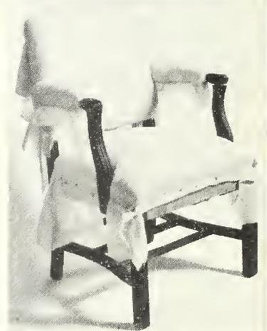
Cut burlap 2 inches larger than seat frame. Attach with #6 tacks around frame. Tack edge rolls to sides and front, keeping flush to outer edge of frame. Cut rubberized hair ¾-inch thick to fit chair seat and cover edge rolls. Stitch in place. Add 2 layers cotton batting extending over seat to underedge of chair. Measure muslin to cover entire seat. Tack under frame. Trim excess.
