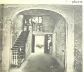
New central hall arch, right, was made from a molding taken of crumbling original.
