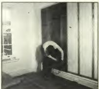
After furring frame is made, panels are nailed in position
