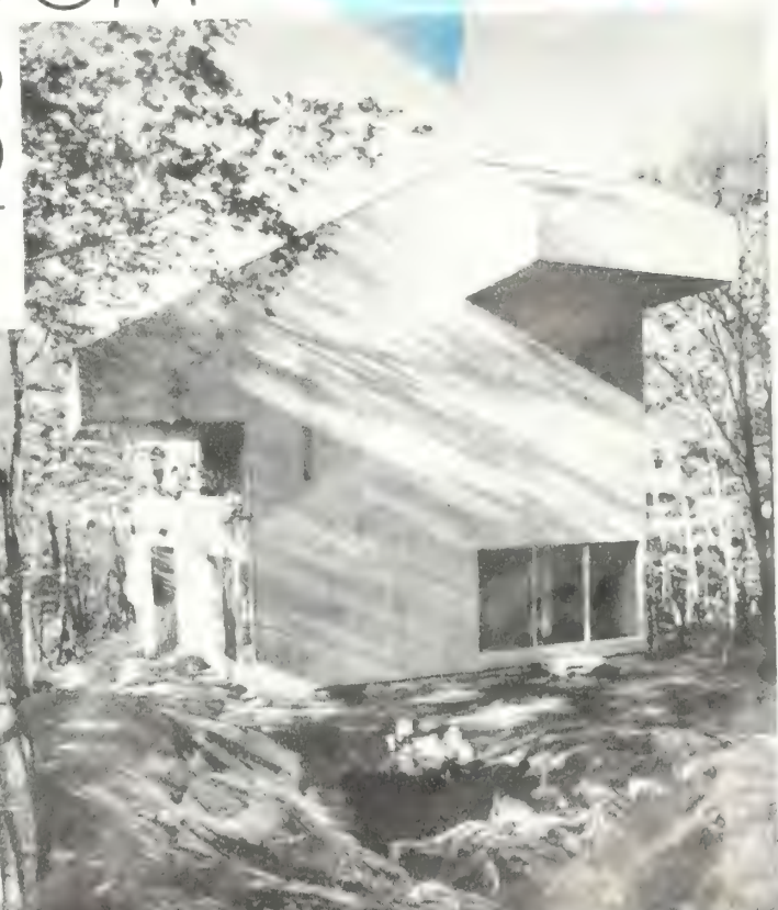
Entrance to house is through sliding glass doors, above, far below high solarium deck. Two story studio at rear, left, has same glass doors used as a window. This 8 by 15 ready-made unit of sliding glass panels, used throughout house, established dimensions of modular forms.
