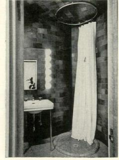
Originally, the bathroom, enclosed in the round brick chimney, was wholly lined with cork except for the concrete floor of the open shower. A few years ago, the walls were resurfaced with leather tiles and the floor with mosaic tile, turning the whole room, in effect, into a shower room. (The guest house bathroom has been supplemented by a sauna designed by the architect, Reino Aarnio.)
