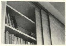
In the guest house, the sliding panels of fabric serve not only as curtains, but as screens for bookshelves and storage. Like the fabric panels in the main house they operate on four ceiling tracks—a custom-installed device that is now available as a standard fixture (page 255).
