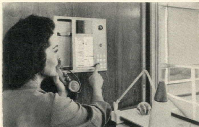
THE SEE-AND-HEAR PHONE is imminent. Two-way television carried by telephone lines will enable you to see your caller on a tiny screen at the top of the control panel, transmit your own image through the eye next to it. Also built into the panel: push-button and automatic dialing, a speaker that relays your voice and your caller's without your picking up the phone.
