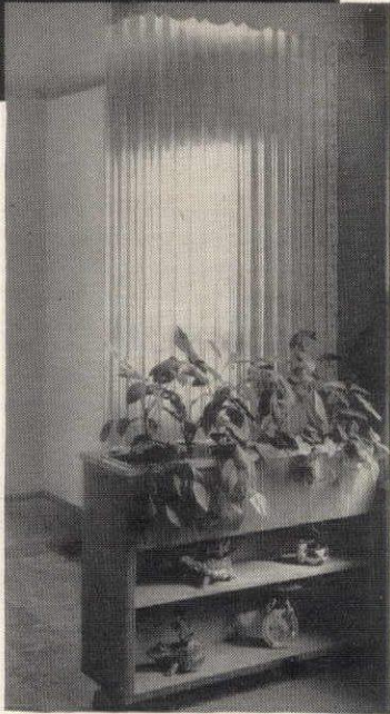
Effective separation of dining room and kitchen with Structural Corrugated glass. Builder, Nordale Realty Company, Milwaukee, Wisc.
