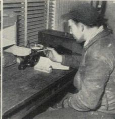
Sample pieces of wood in kilns are carefully weighed to check moisture
