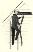
Loose fill insulation is lightweight, can be applied to walls and attics of houses, old and new.
