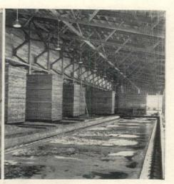
Cooling shed at discharge end of kiln battery. Lumber is held here to equalize at normal use temperatures.
