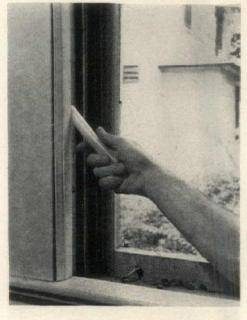
5. When the window is open, trim off all of the still sticky particles and edges of paint with your knife. It's a good idea to rub candle wax thoroughly along all of the sliding portions of the casement to make future raising and lowering smooth and easy.
