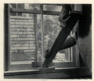
4. The window may now be loosened, but you find you still can't raise it. This calls for the fulcrum method. Screw a strip of wood to the lower edge of the frame and another to the window ledge. With a length of wood serving as a lever, work gently up and down in a prying motion until the window is raised. Fill screw holes with plastic wood afterward.
