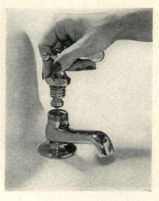
3. Now turn the faucet handle in a clockwise direction just as though you were turning on the water. Keep turning until the central core, which is called the spindle, is completely unscrewed. Lift spindle out of the body of the faucet.
