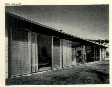
Alternating plate glass panels and glass jalousies form a ventilating window wall the full length of the house, giving all rooms a view. A simple crank turn opens jalousies for any degree of air desired. Architects: Twitchell & Rudolph.
