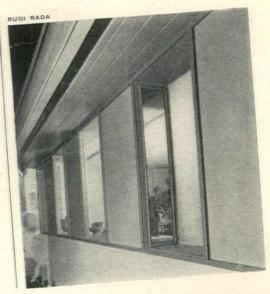
Vertical louver windows, lining recessed sections of the front wall of the house, admit light and air but shield interior from street view. Storage cabinets may be built underneath on the inside. Architect: William E. Kittle.
