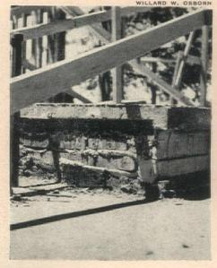
Foundation of house is a concrete slab with waterproofed, insulated crawl space below.
