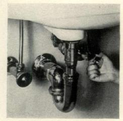
1. First, turn on the leaking faucet and let the water run. Next, turn the valve beneath the basin in a clockwise direction until the water ceases to flow from the open faucet. If no shut-off valve is there, you will need to close the main water valve in the basement, or utility room of a basementless house.
