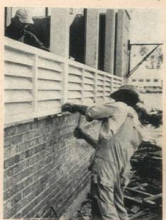
Louvered panels under fixed panes of insulating glass ventilate the bedroom wing.
