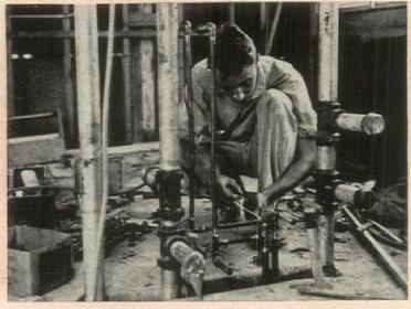
Location of all kitchen equipment is precisely planned. Plumbing pipes go in concrete floor, set position of sink and laundry.
