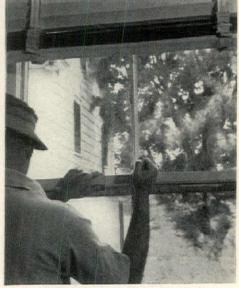
1. Tap gently all around each frame with the side of your hand—this method sometimes works. But don't ruin a good hand on a stubborn frame. Another caution: don't hit so hard that you break the glass or the frame. Be especially careful near the center of the window where the casement does not brace the frame.
