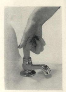
6. Before replacing the washer, feel down into the open body of the faucet. If the small brass ring at the bottom is rough or cut, it needs to be smoothed with a faucet reamer or it will soon wear out a new washer and cause another leak. Full directions will come with the reamer, which you can buy inexpensively at a hardware store.
