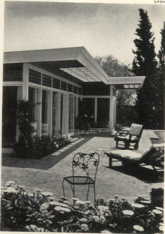
Egg-crate overhang shades south windows from overhead summer sun and from glare but lets desirable winter sun in.
