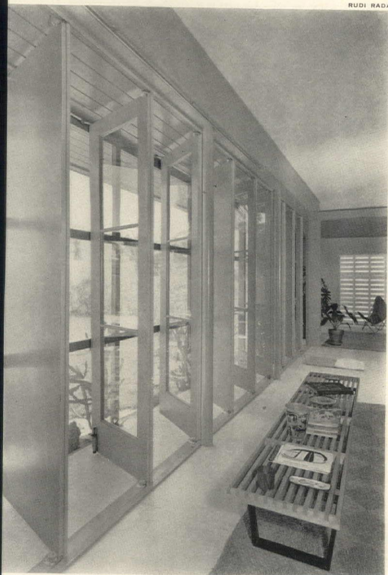
Sun, air, rain are controlled here by roof extension, by outside screen, by doors that open together like louvers.
