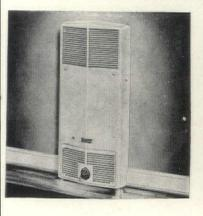
"Saf-Aire" gas heater is light enough to lift by hand, fits snugly into any outside wall, produces ample heat for rooms 12' x 18' and is proof against fire, explosion and asphyxiation hazards. Heating fumes are vented outdoors without costly chimneys or noisy blowers. Outside air is drawn in for combustion, thus preventing condensation indoors. \$100, installation extra. Heating Research Corp., Muncie, Ind.
