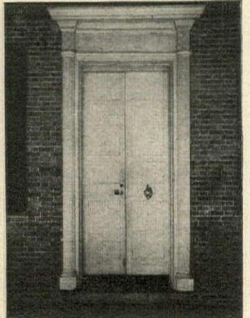
Reeded half columns topped by diapered carving and dentil moulding flank Beckford's dignified double entrance doors
