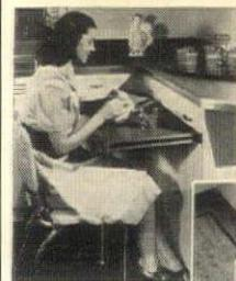
**SLIDING TABLE** provides secondary work height. Slides into base unit when not in use.
