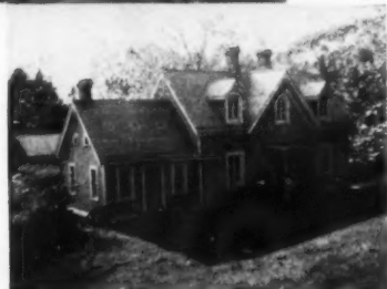
FRONT VIEW BEFORE AND AFTER
