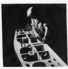
For pattern, Swiss cheese has nothing on the huge sheets of plywood which are shaped to make framework of glider, Here a workman smooths edges for inspection.
