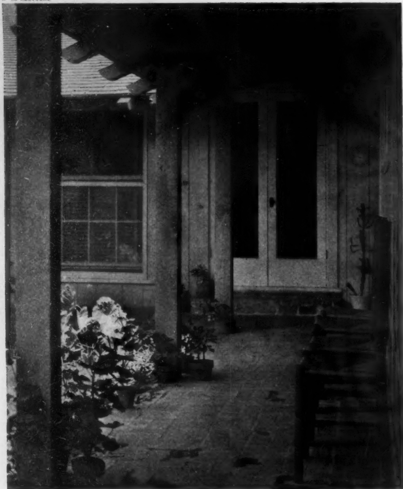
Wide, gently sloping eaves, supported on sturdy posts, shelter the brick-floored terrace which runs around two sides of the walled patio and provides a pleasant place for outdoor dining.
