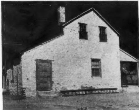
OLD WHITE STONE HOUSE, FREDERICKSBURG
