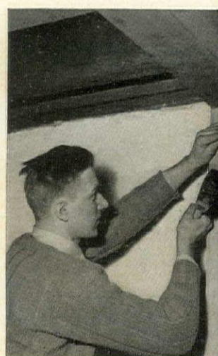
3. Stout studs are spiked to new beams which have been installed to reinforce existing ceiling
