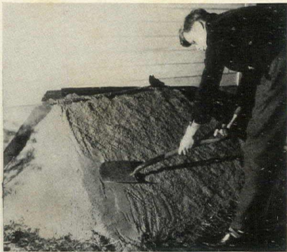
5. Sand, to an average thickness of 3' is piled against the wooden form, which is protected from the weather with roofing felt. Cover sand with turf
