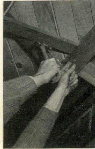
8. To strengthen ceiling add supplementary joists and brace between them with sections of 2" x 4" lumber
