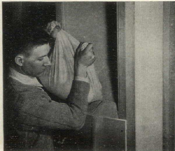
10. Protective filling of sand is poured between wallboard. Sections are nailed to end of wall as it is filled up. Paper sand bags could also be used
