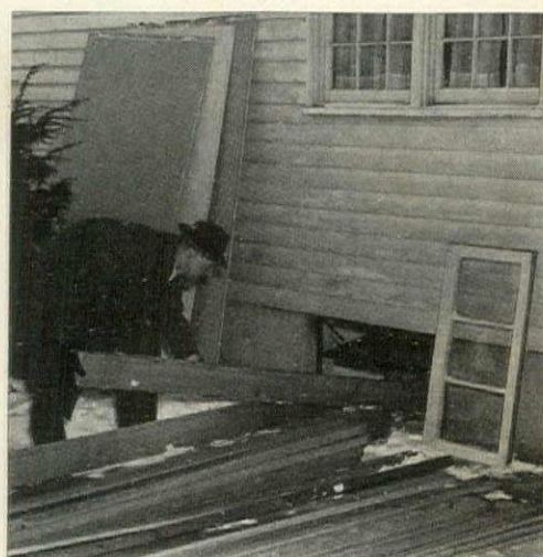
2. Heavy timbers (6" x 6") are slid into the cellar for reinforcing existing ceiling construction in case house should collapse
