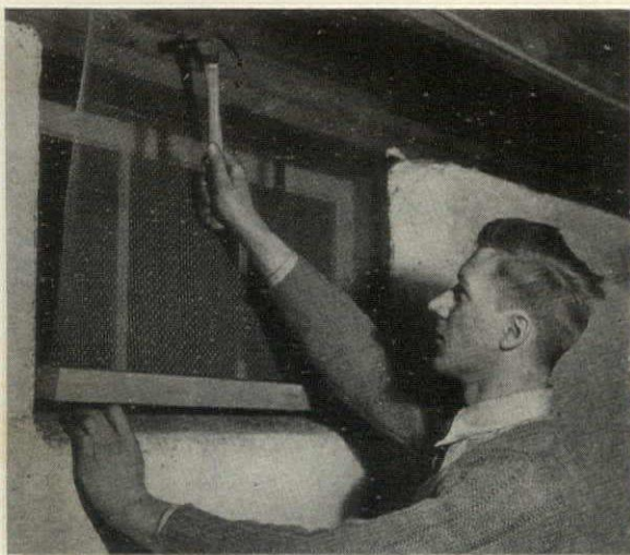
5. Protection from flying glass, splintered by con- cussion, is achieved by hanging wire mesh over window. A 2 x 2 at bottom of mesh keeps it in place
