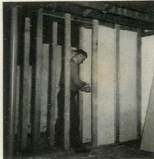
2. First step is the construction of a protecting wall. Sections of wallboard are nailed to the studs, reinforced with wire
