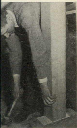
for a secure base, reenforcing are nailed to large square s placed on the cellar floor
