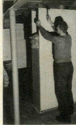
3. Sides of protecting wall completed and sand is poured between the wallboard sections
