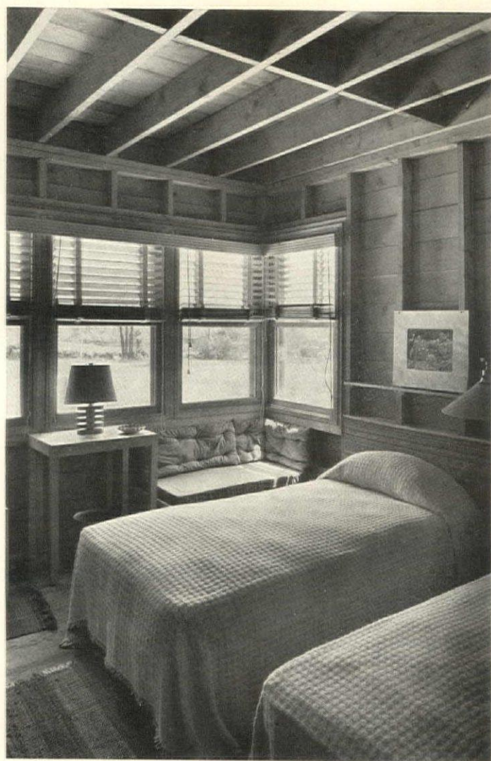
The first floor bedroom. To maintain the rhythm of solids and voids, the architects arranged the rafters to coincide with the studs. The sheathing is Douglas fir, to match the other woodwork
