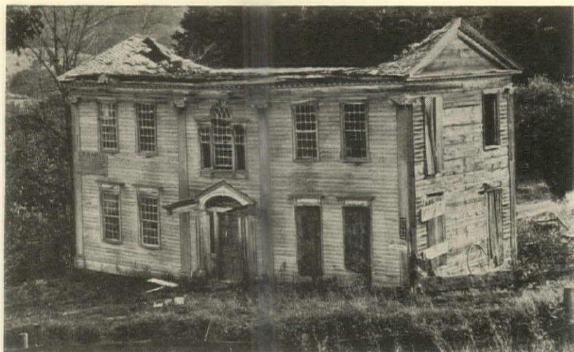
Before restoration: The Elisha Morgan house, badly dilapidated, still showed traces of its fine late 18th Century detail. The roof had fallen in and the beams rotted, but the Palladian window over the door had not lost its dignity
