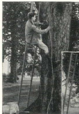
After Bartlett has completed a Lightning Protection installation, the whole tree becomes, in effect, a giant lightning rod which not only dissipates "ground charges" but carries all bolts harmlessly down the trunk and into the ground.
