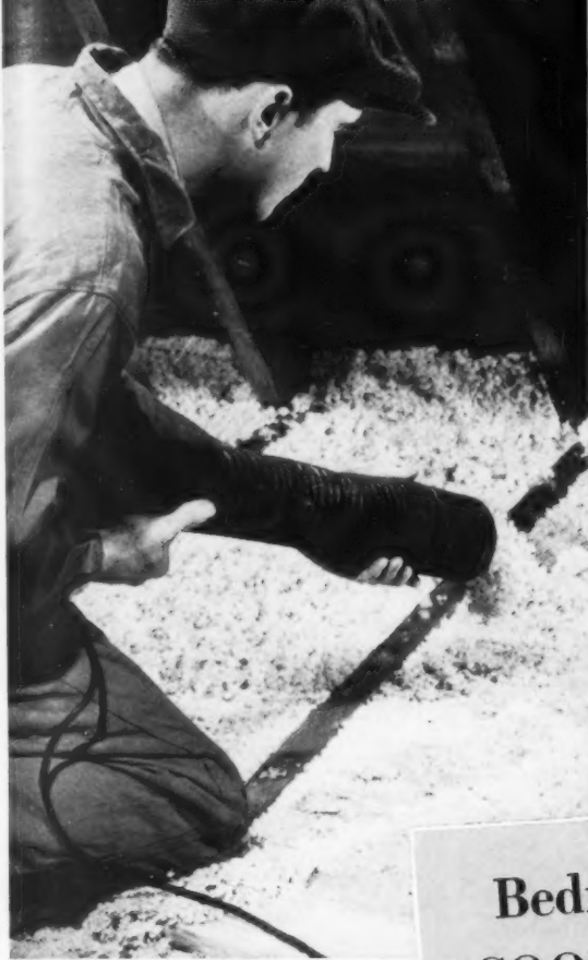
"Wool," MADE FROM MELTED ROCK, is blown into the hollow spaces between your attic and your upstairs rooms, making an invisible barrier against heat.
