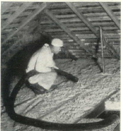
J-M Home Insulation is quickly and simply installed
