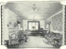
In the Reaves' home, Armstrong's Corkboard is used on all the exterior walls and second floor ceiling for insulation against heat and cold, and on the interior partitions and first floor ceiling for sound deadening. Plaster is applied directly to the corkboard
