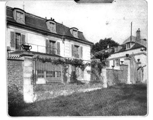
The shallow, curve-topped dormers in this house at Viroflay, France, are partially recessed by the projection of the eaves beyond their base, the eaves running in a continuous line. An iron bar carries across each window the intersection line of roof and dormer
