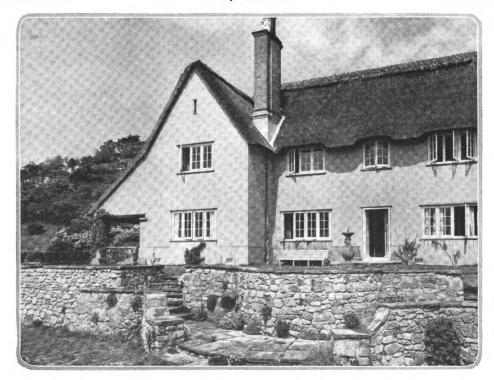
One of the great beauties of thatching con-sists in the ease with which it can be fitted to an ir-regular line on the ridges or eaves. Oswald P. Milne was the architect
