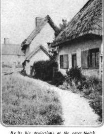
By its big projections at the eaves thatch By its dig projections at the cases that it roofing is able to protect the walls from the weather. The material on these cottages at Rye, England, is straw
