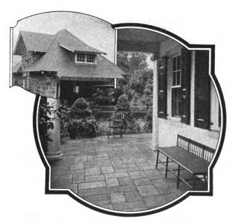
The diversified uses of slate are illustrated by the three photographs. Slate roofs are economical for cottage or mansion. Slate walks and floors are most serviceable as well as beautiful, while for sanitary usage such as sinks, toilet partitions and table tops, slate is unsurpassed.
