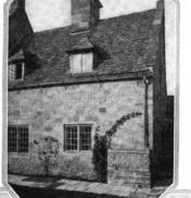
The corner of a house in Gloucestershire, England, showing leaded casements used in dormers and the hipped roof construction in their covering. Sides and roofs are of slate
