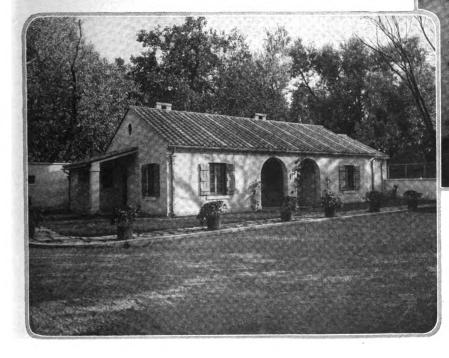
In the gardener's cottage, with its graceful double arch and splendid proportions, can be seen the effectiveness of the method used in laying the tiling. One row of flat tiles is laid between every four vertical rows of half-round tiles, giving an unusual texture to the roof
