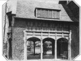
The half-timber work, with brick nogging, is ruggedly wrought of oak, and has been left to weather without finish of any kind. Rough slates, and the random color and texture of clinker brick add to the interesting play of the natural textures of natural materials
