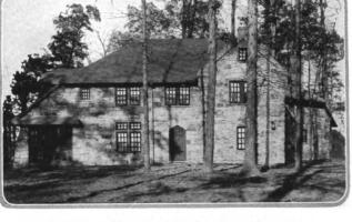
A stone house of interesting roof-profile, using a "Barrett Exer-lastic" slate-surfaced as phalt shingle. Gray, dull red and dull green are the colors in which these shingles are made
