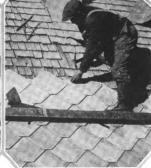
form apparently hexagonal units, are being placed directly over an old wood shingle roof
