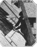
Laying "Flextone" asbestos shingles over an old roof, the roofer uses beveled strips of pine to make an even surface
