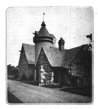
In addition to its use in the roofs of this group, slate has been made to form the circular ledge of the pigeon runway on the tower
