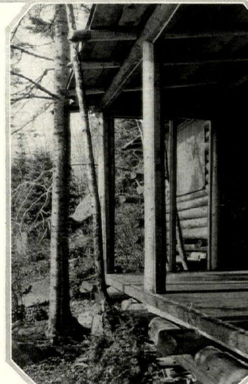
Below: The front wall and porch of a cabin nearing completion, with the framed openings temporarily braced. Two cabiners, in the other picture, are rolling a log into place for the roof
