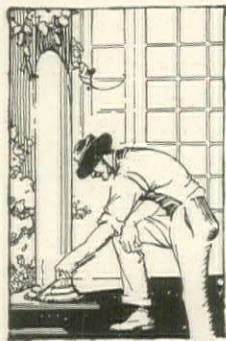
Rot and decay start under porch columns, porch posts and flooring, exterior siding, eaves, gutters, door and window frames, rails, roof or side shingles, mud sills—wherever there is exposure to earth, air or water.
