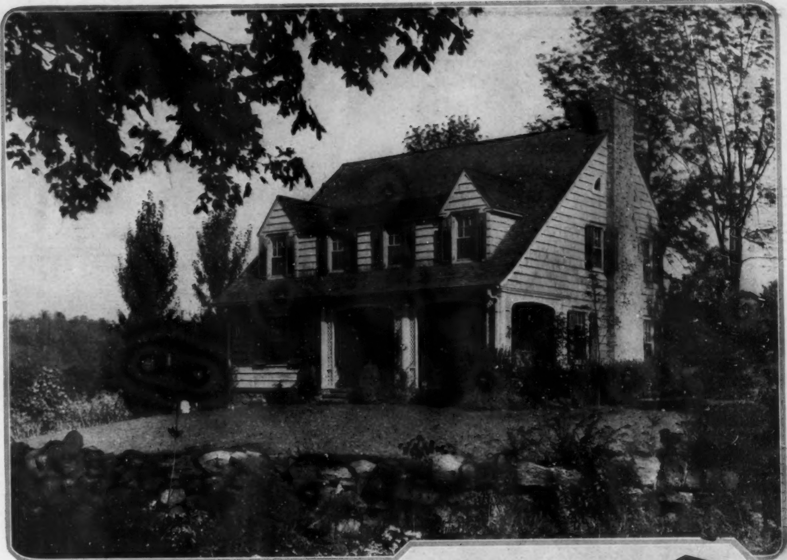
From the rear is another view of the valley. Here is the dining room and the porch, with its lattice panels. This is glassed in winter. The dormers upstairs are joined together by two other windows, giving more space in the chambers
