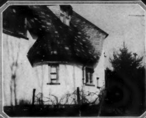
This rear view shows the flare of the roof to cover the laundry extension
