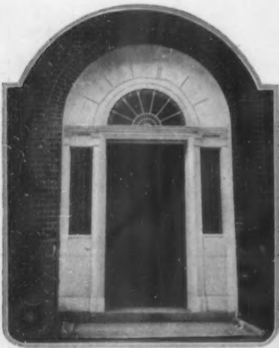
A splendid use is made of wood panels and a fan light to fill the arch of this door. This and the other six doorways are in England
