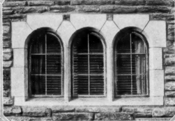
From the outside Venetian blinds furnish an interesting diversity of line
