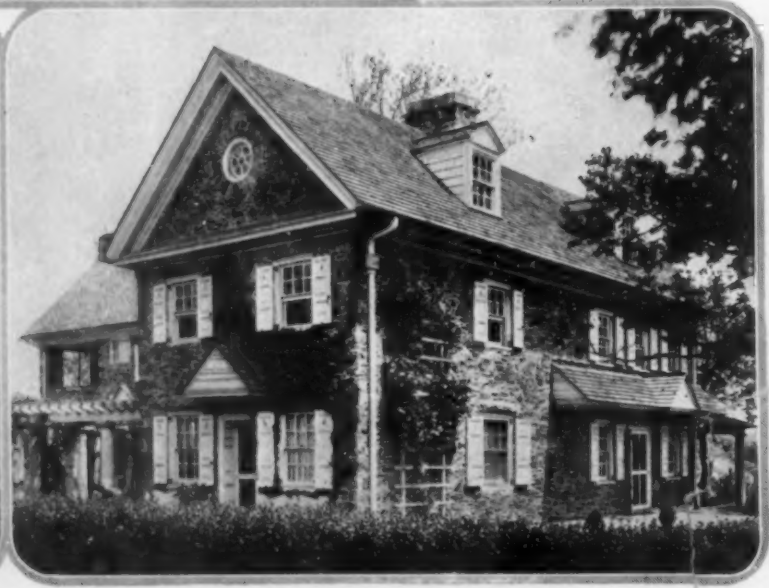
"Wynnestay", Philadelphia, has the Pennsylvania Colonial characteristics—field stone walls, wide eaves, pent roofs over doors
