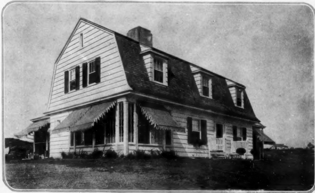
The gambrel roof type is a favorite Colonial style because it is pleasing to the eye and affords the greatest possible space for the outlay. Aymer Embury II, architect
