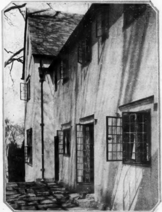
Leaded, metal casement windows and doors maintain the English atmosphere on this façade. The terrace is paved with flags laid irregularly and allowing space between for grass, which softens the effect. One is especially struck with the silhouette possibilities of these casement windows
