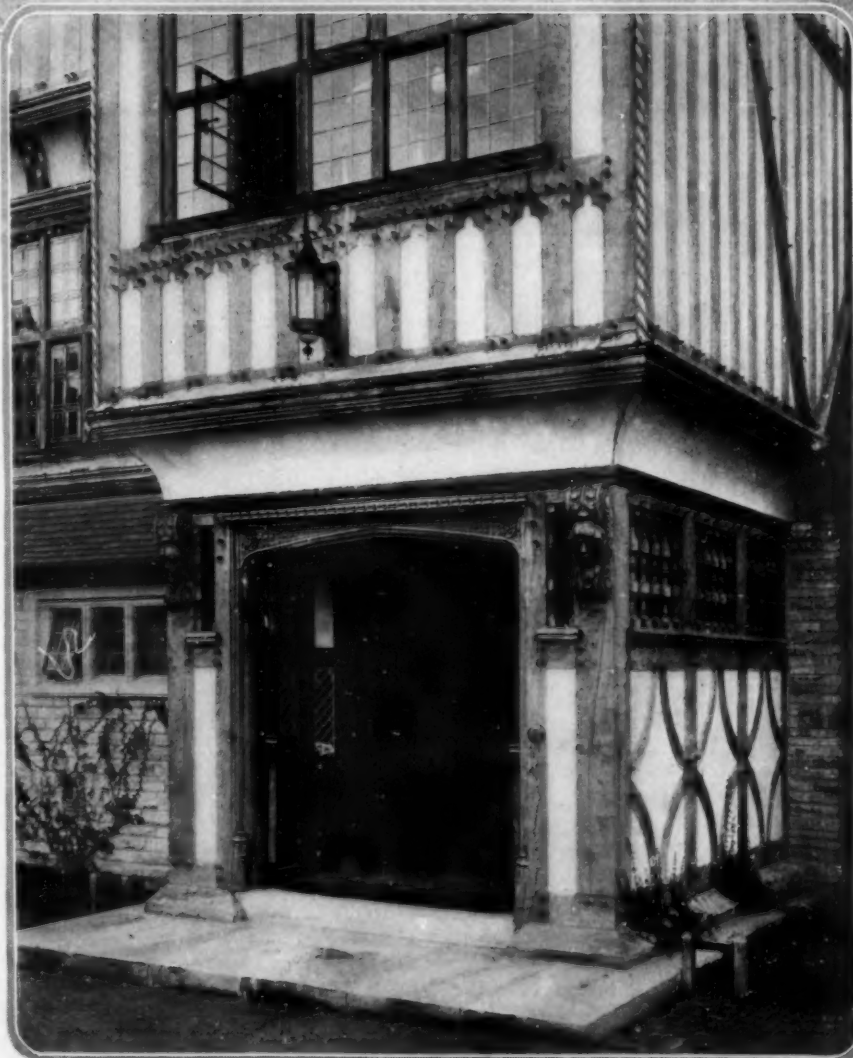
The carved and turned enrichment of the house door details is a strong asset in fixing character to the whole composition. It is enrichment concentrated where it will prove most effective. The wood is oak. The leaded metal casements and wrought iron lantern are in harmony with this carving and half-timber
