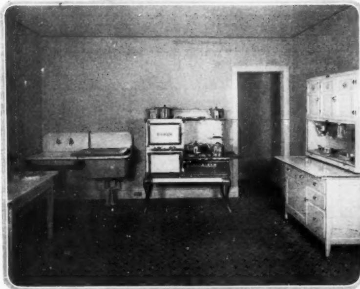
Inlaid linoleum for the floor, painted walls, a serviceable cabinet and stove and sink properly placed make this an ideal small kitchen
