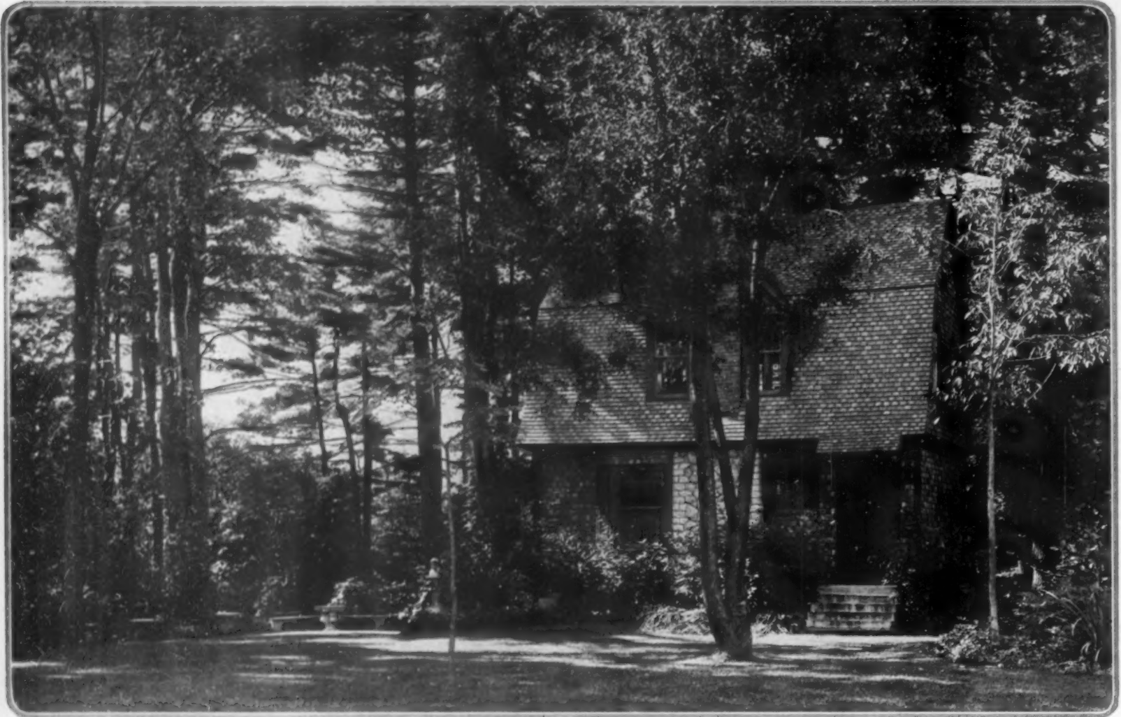
Mr. Cable's study is a fieldstone Dutch Colonial building, set in a grove of giant trees. Wide lawns stretch before it. To one side is a little grouping of stone benches that form a garden resting place
