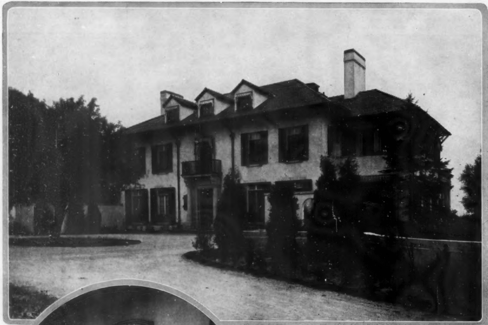
A walled-in garden on one side and a terrace wall give formal approach to the house and enclose the turn of the drive. The house is Italian in feeling. The material is stucco, the roof is tiled.
