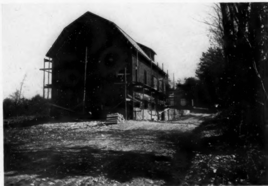
It was a cross between a city stable and a country barn. The first floor is for the horses and cows, second for carriages and wagons and the third a hay loft. Cost complete, $3,264.96
