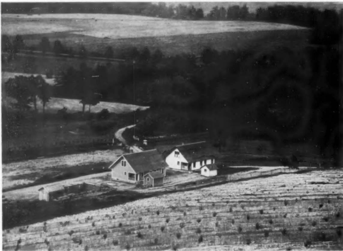
The bungalows for the farm hands were situated near the main road, the first serving as a lodge. Two were built and the foundations laid for a third. Complete cost, $4,775.41
