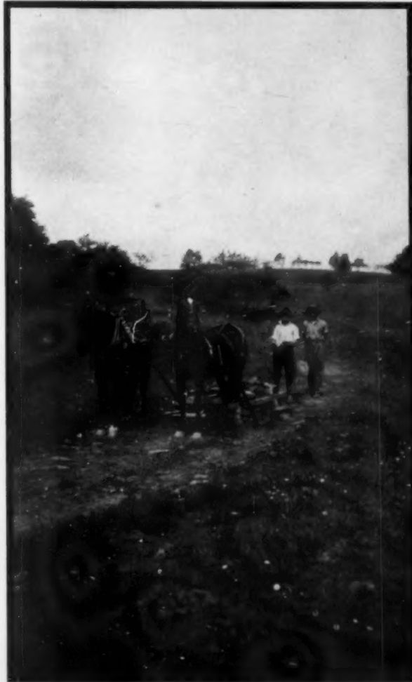
The orchard land was covered with stone, and this was hauled to build the road; the cost amounted to $491.80
