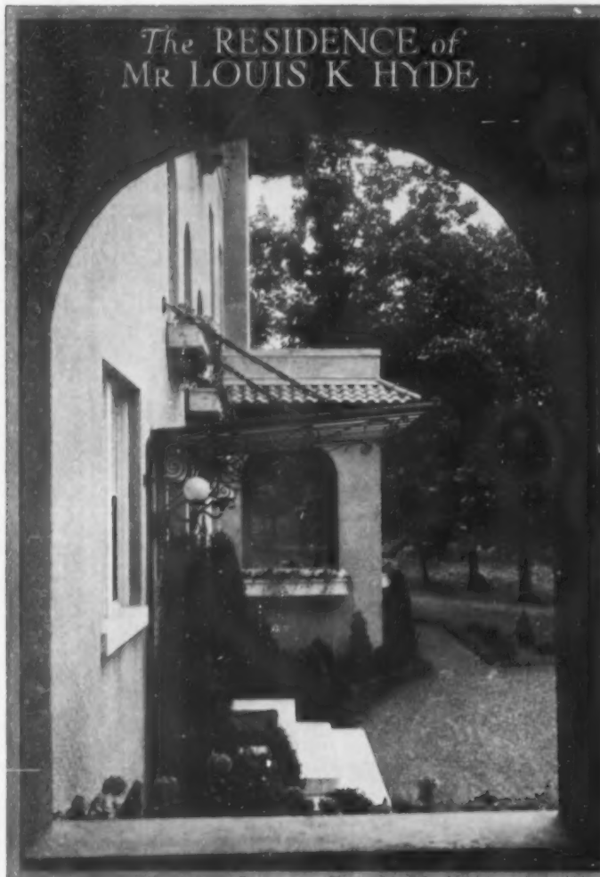
Situated just back of Plainfield, New Jersey, "Oakmont" is approached by a beautiful drive winding up the Watchung Mountains. The Italian architecture of the house has been modernized and adapted to American living requirements. Spanish tile of variegated dull green and red gives the roof an appearance of old copper. F. B. and A. Ware, architects
