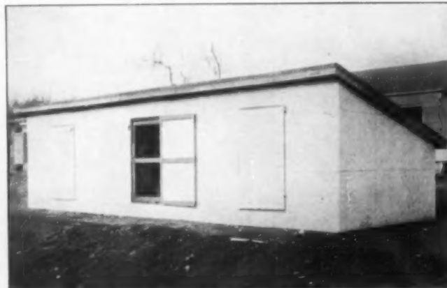
Stucco board cuts the cost of construction at least 10 per cent. This material, which comes in squares and is nailed to the frame, is rapidly growing in popularity
