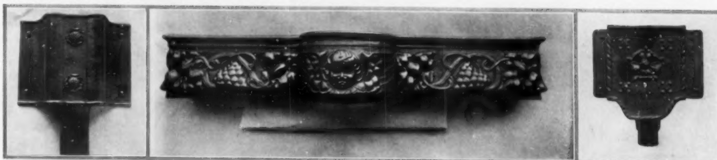
Though severely plain, the head adds finish to the down-pipe
