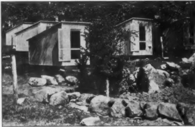
Fresh air colony houses of the shed roof type may be constructed at an average cost of fifty dollars for fifty hens or may be purchased ready made
