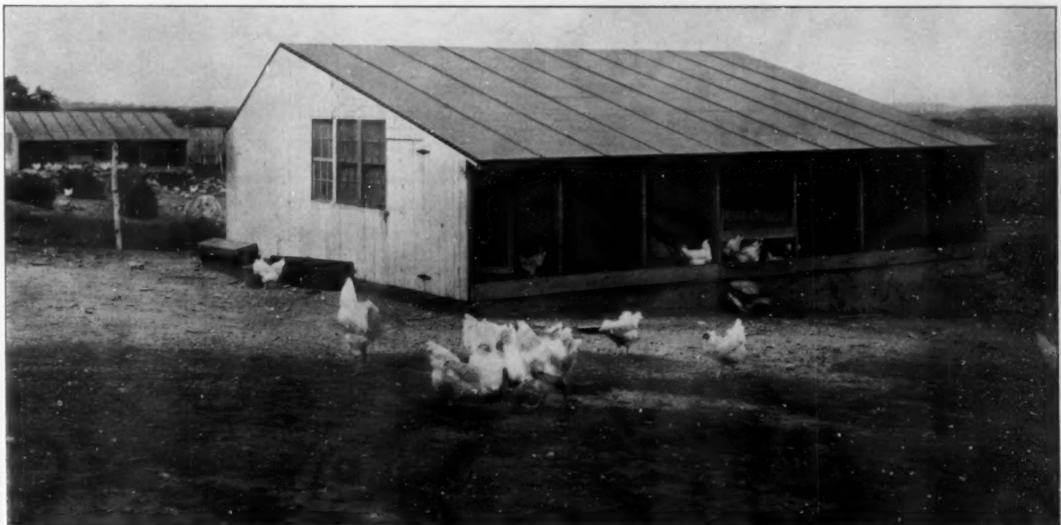
Still in common use, the Tollman type of house, large enough to accommodate three hundred hens, may be built for about $275
