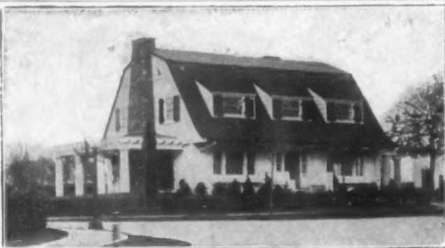
Stained with Cabot's Shingle Stains Forman & Light, Architects, 40 Cedar Street, New York
