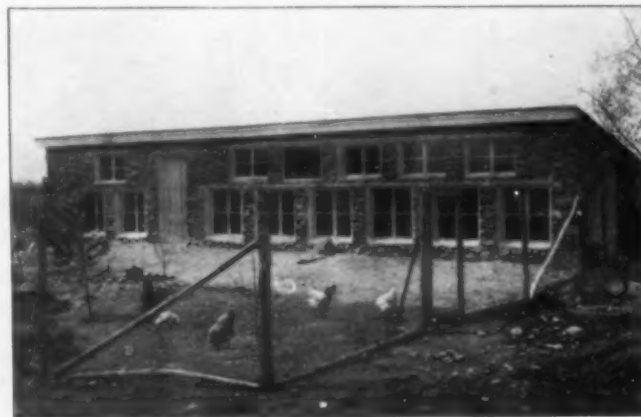
Field stone may be employed effectively when one's residence is of the same material. Naturally such a building is more expensive than a frame house of the same size
