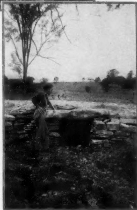
Meadow rivulets are lively creeks in the spring, hence the culverts with heavy stone caps
