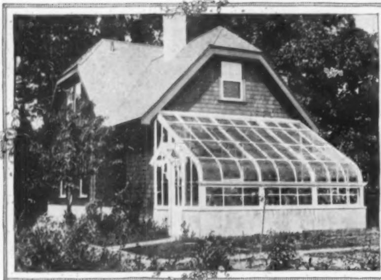
This type of lean-to attached to the southern exposure of a house in Massachusetts, opens both indoors and out and consumes comparatively little fuel
