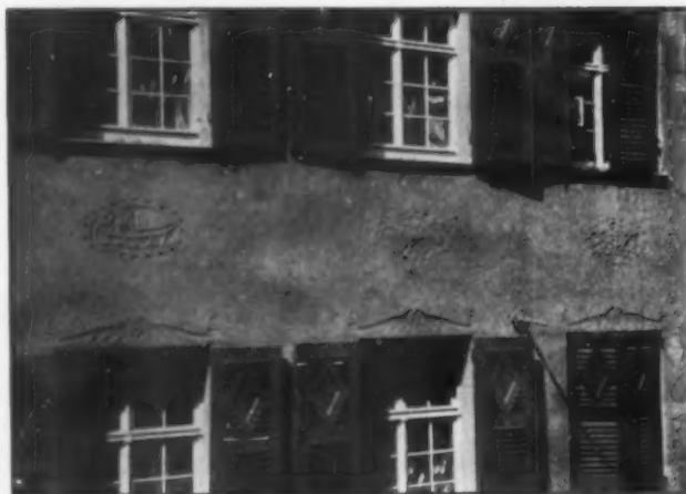
Sgraffito ornament in browns, greys and yellows, are used on all the buildings. The shutters are carved with decorative designs and painted a dark green
