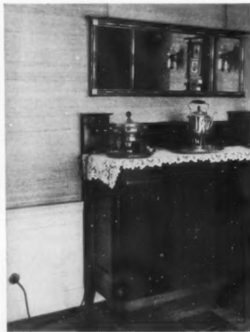
A baseboard outlet for gas will be found useful in the dining-room
