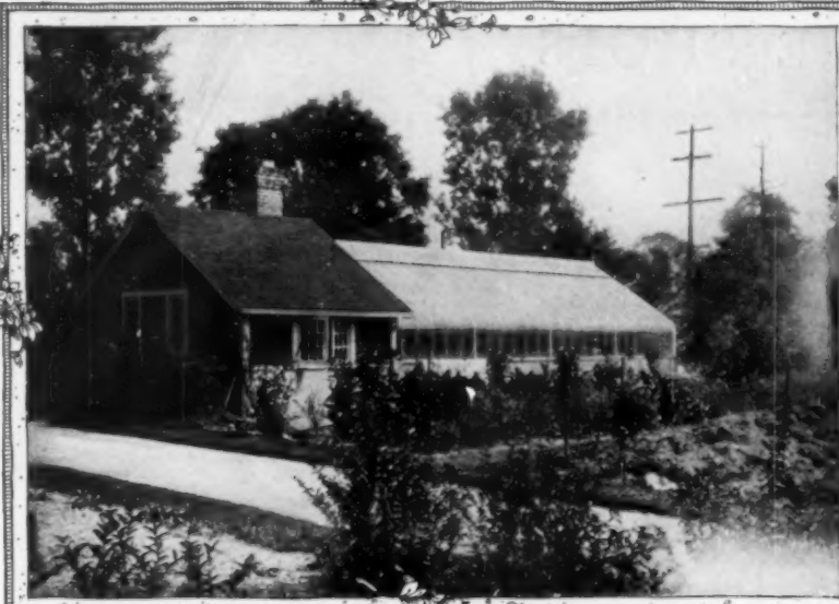
No country place is complete without a garage and a greenhouse, and the simplest plan is to link them together and have a unit heating plant
