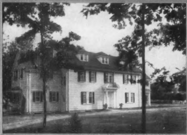
A wood house: wood frame, roofed with white cedar shingles and the walls covered with red cedar painted white, a combination suitable to a rural environment
