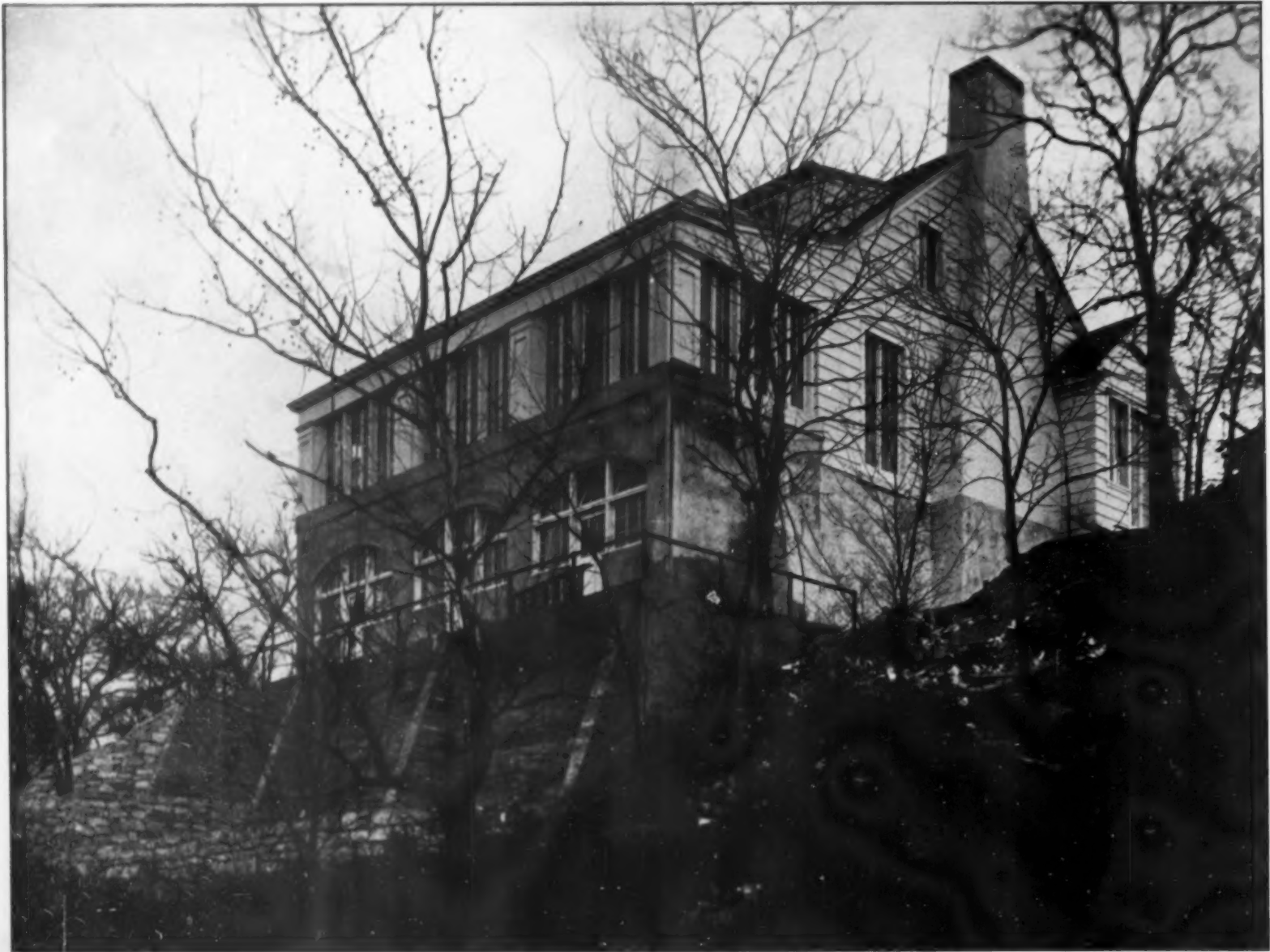
The main factor in construction expense was shoring up the foundations, as the lot was on the edge of a steep hillside. It gave, however, a diversity of levels to the rooms and added interest to the interior
