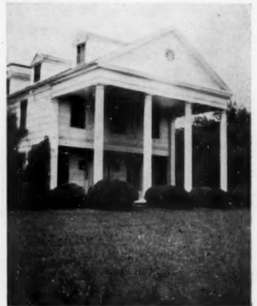
By introducing box, a Southern Colonial portico at the Breese house instantly assumed the verisimilitude of antiquity
