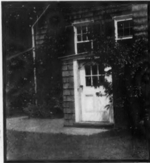
Entrance to the cellar through an outside vestibule establishes a separate, private and convenient connection between both parts of the house
