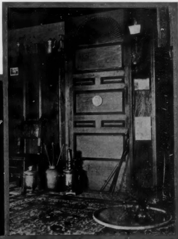
Mainly junk—here in the living-room is a discarded fan-top door; the wainscot is made of old shutters
