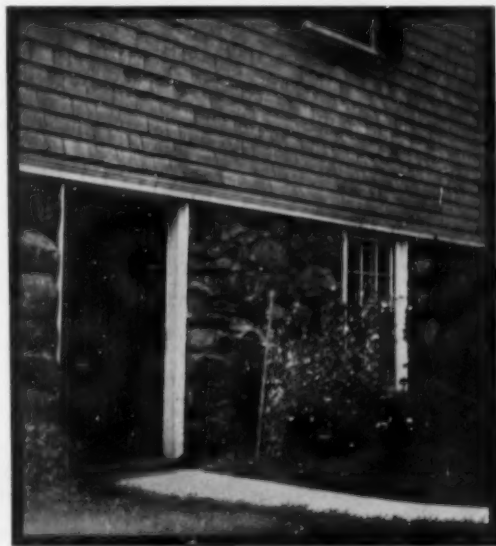
The most practical of all cellar entrances is the vertical door without areaway
