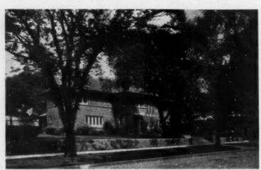
A house in Oak Park, Ill., built of brick with limestone trimmings, where the straight lines harmonize with those of the street. Spencer & Powers, architects
