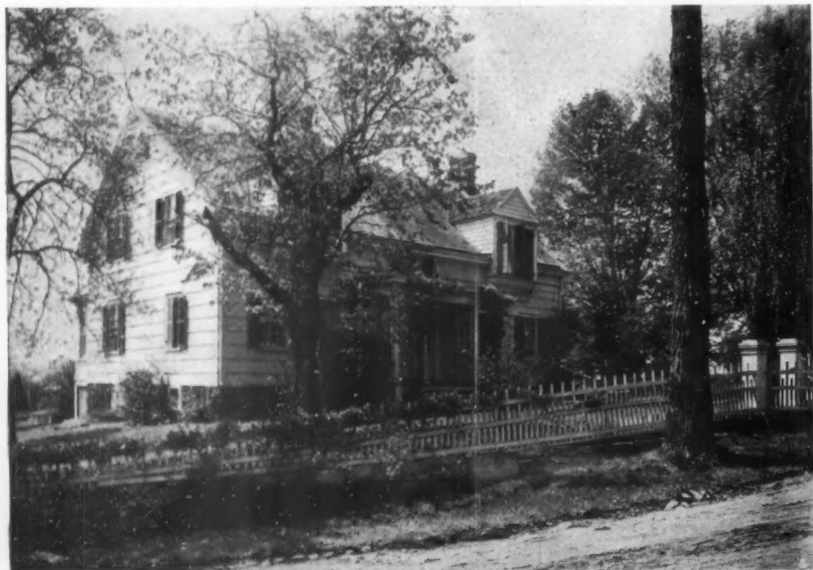
One of the solutions of a common problem. In old houses the second-story windows are near the floor, under the cornice, and must be enlarged to make the bedrooms livable
