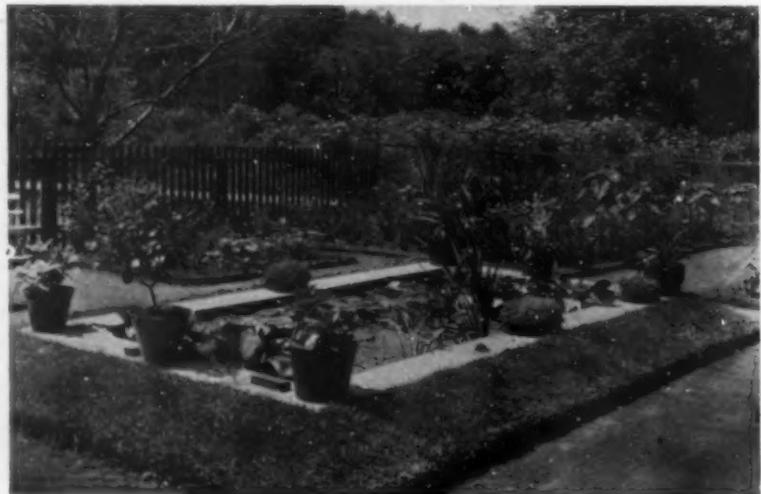
A cement pool must be drained in winter or have sloping sides that will not resist the ice
