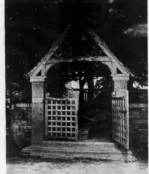
A quaint roof shelter of large flat tiles protects the sturdy, centuries-old oak timbering in posts and brackets
