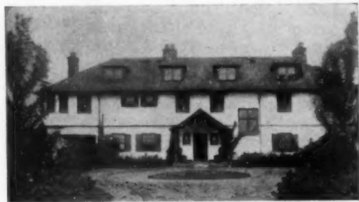
The home of Thomas Shields Clark, sculptor, Lenox, Mass. Wilson Eyre, architect
