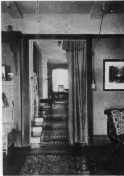
An unusual and ingenious arrangement of lighting fixtures, where the bulbs and cords are suspended from wooden arms on the side wall woodwork
