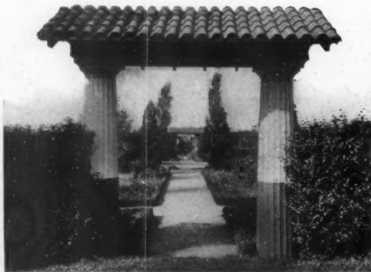
An entranceway of "Chelton," near Jenkintown, Pa., Mr. Wilson Eyre, architect. The columns are roughcasted in maroon and buff, the roof of red tiles
