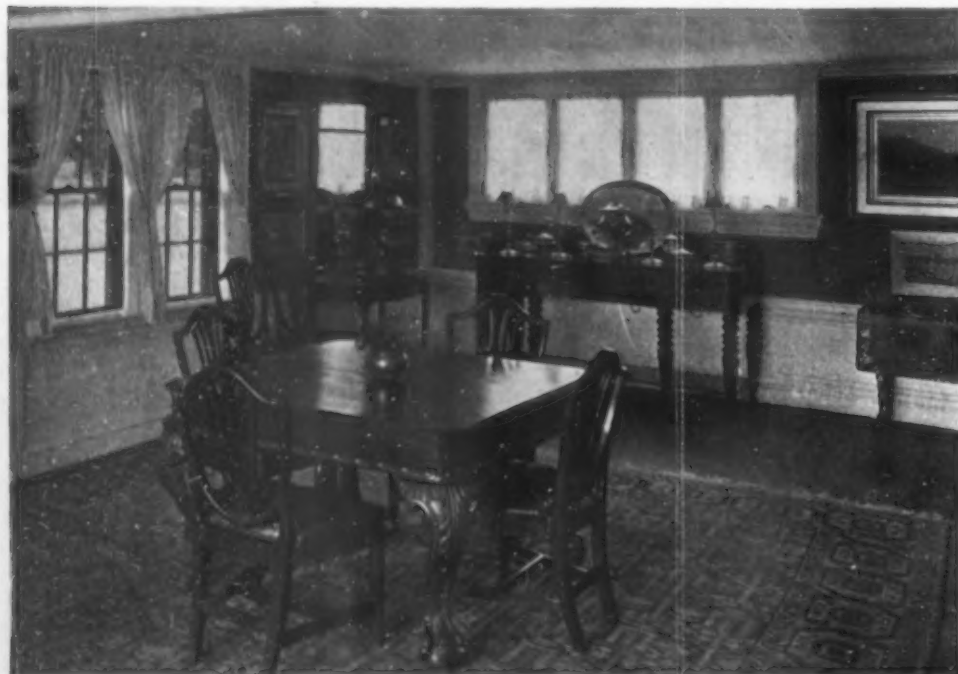
A very clever semblance of wainscoting has been secured by painting white the plaster between baseboard and chair-rail, and running the upright wood members across
