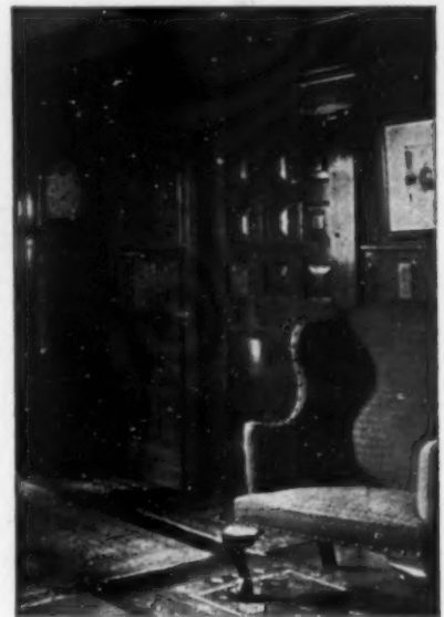
Strip paneling in red oak that has been given a soft brown finish without gloss by means of oil and wax. The wall above is covered with a green burlap. C. E. Barott, architect
