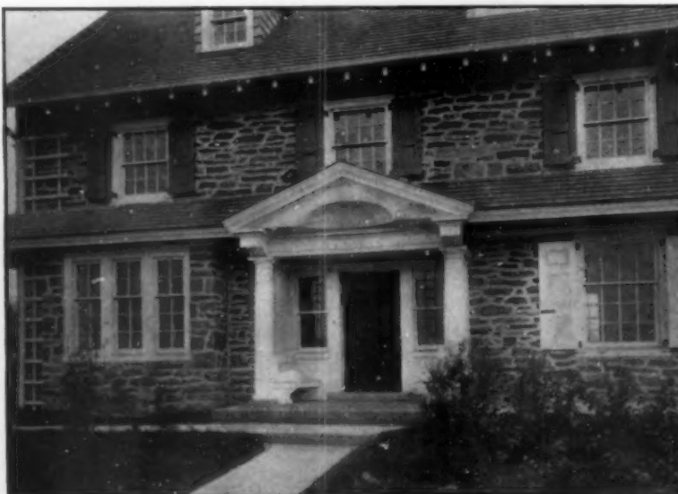
Two built-in seats flank the front door on a brick-paved terrace that is carried around from the porch
