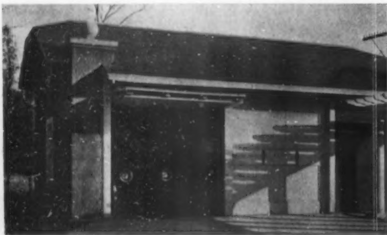
The folding door is an ingenious feature of this Western garage, designed by Tallmadge & Watson, architects
