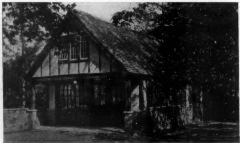
An abundance of windows make the interior of this Syracuse garage a convenient repair room. Alfred T. Taylor, architect
