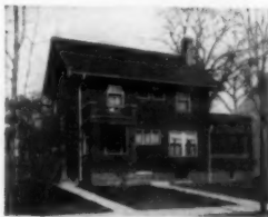
A No. W-25 IDEAL Boiler and 500 ft. of 3/8-in. AMERICAN Radiators, costing the owner $245, were used to Hot-Water heat this cottage.
