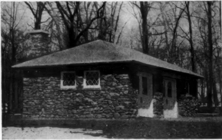
Rough field-stone walls are backed up with reinforced concrete, and the roof is of the latter material
