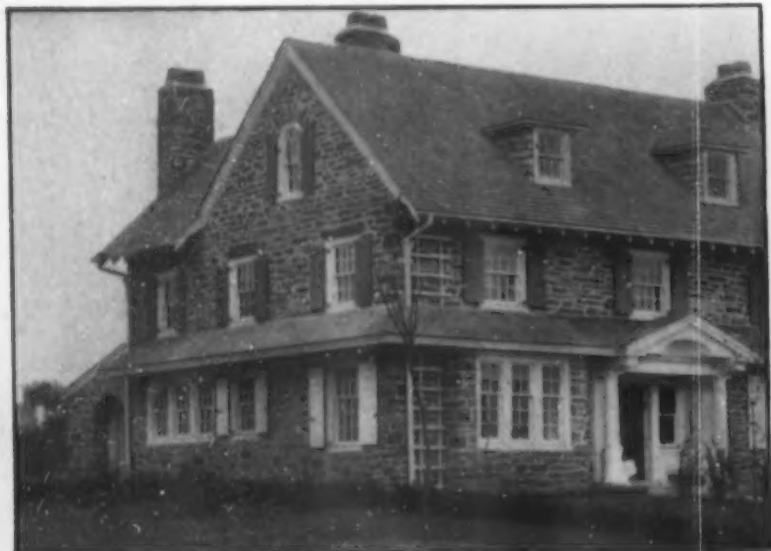
The shingled roof sheltering the first-story windows is a feature commonly called the "Germantown hood"
