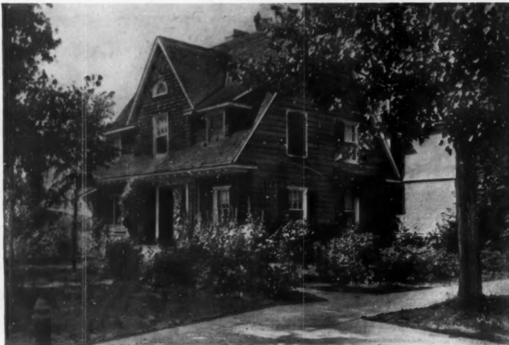
The house is placed near a front corner of the 54 x 160 ft. lot, but with its entrance at one side and its living-rooms at the rear or garden front
