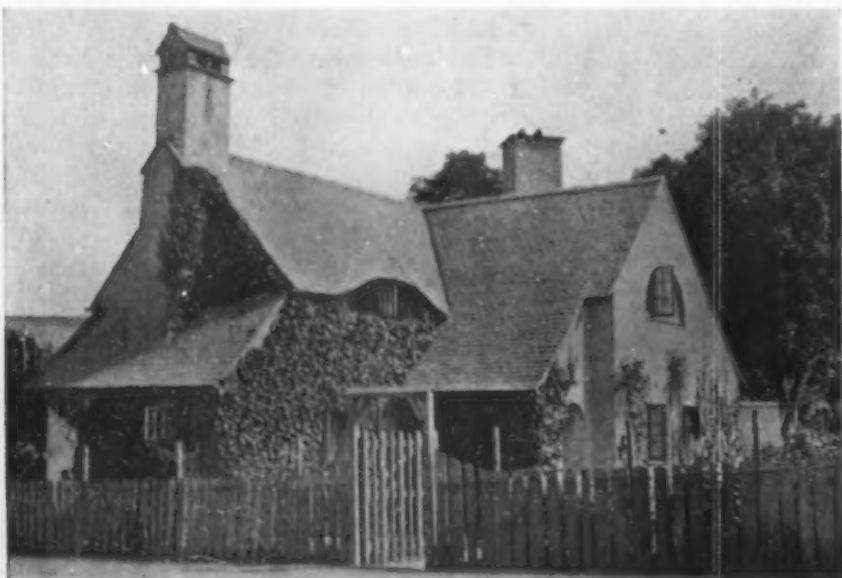
"Bolnhurst," Llanfairfechan, North Wales, is an excellent example of the possibilities the English plaster house possesses for picturesque mass. H. L. North, architect
