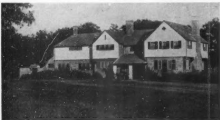
The use of shingles as a base, with plaster above, marks this informal country house at Hamilton, Mass., for Messrs. A. L. and F. D. Cochran. Parker & Thomas, architects
