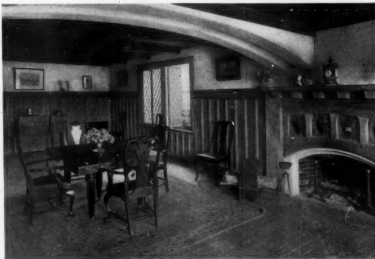
A simple and effective wainscoting of battened oak boards
