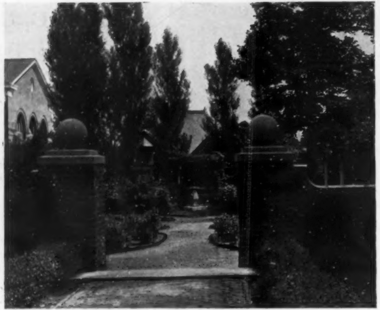
Brick piers are more costly, but also more durable than wood work; the caps may be of stone or cement
