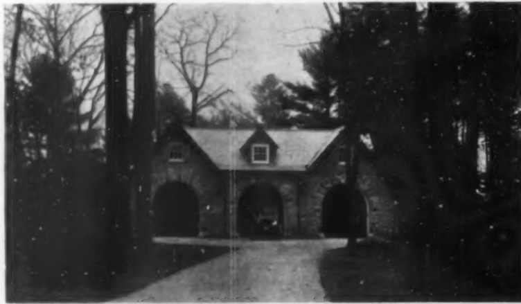
A garage at Chestnut Hill, Mass., with wash-room and repair room back of the car room on the central axis, permitting easy handling of the cars entirely under shelter
