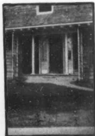
A wide overhang of the roof shelters the main entrance
