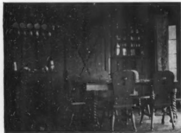
At the right the cupboard is built in so as to be flush with the woodwork
