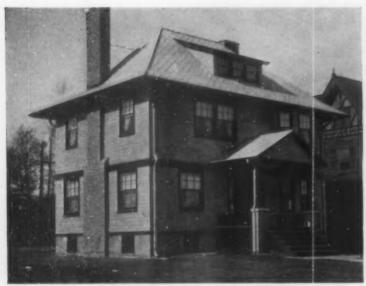
The asbestos shingle is a modern fireproof roof covering handled very much like slate
