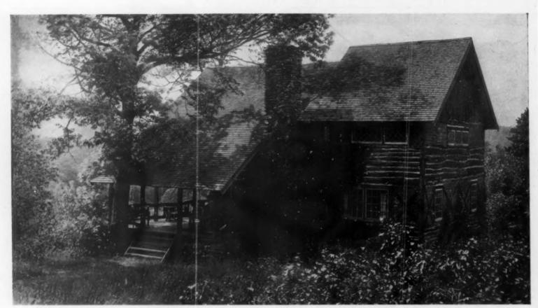
The outside cuts from chestnut logs were nailed to an ordinary stud frame, the chinks being filled with cement on wire mesh
