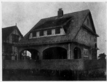
Wood shingles are the most common roofing material. The rounding off of edges is called "weaving"
