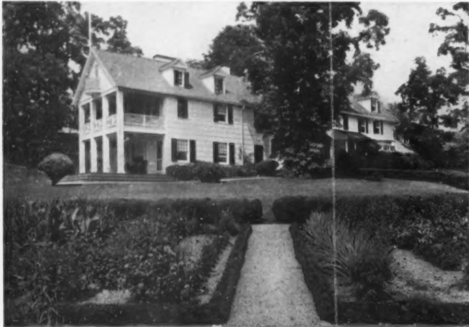
A modern house along Colonial lines with walls of hand-riven shingles painted white. Few things contribute so much to the old-time atmosphere as well-grown box
