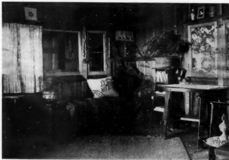
In this $1000 bungalow the upright boards of the walls were merely battened inside and out between the studs, then stained
