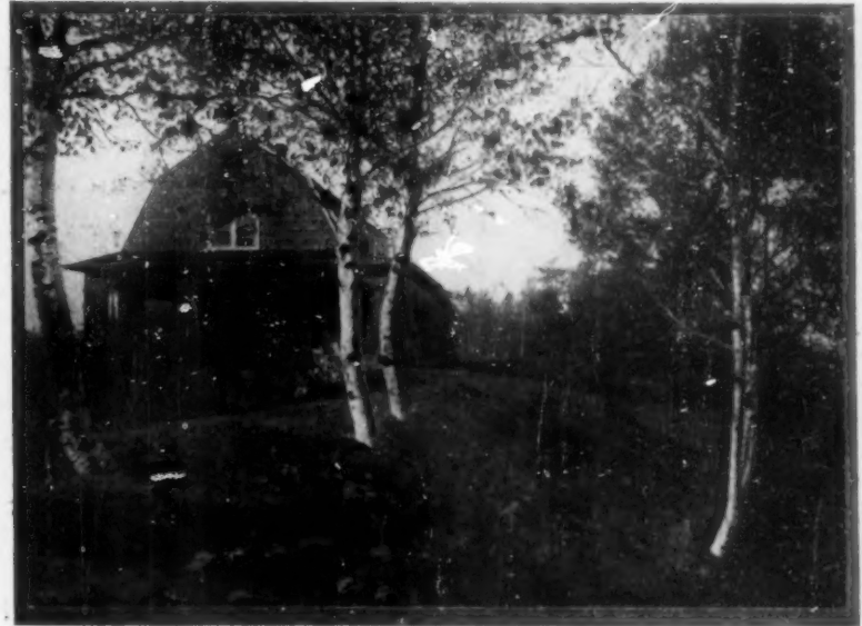
A wide porch extends across the lake front and one end of the Lodge and forms the outdoor living-room throughout the summer months
