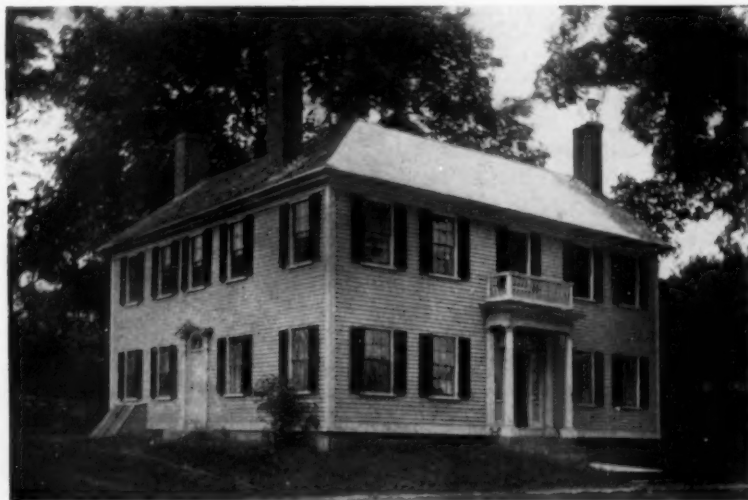
In New England the materials used were clapboards and shingles in contrast to the Southern brickwork
