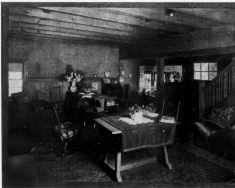
In the living-room the second floor joists have been allowed to show in all the honest ruggedness of straightforward construction
